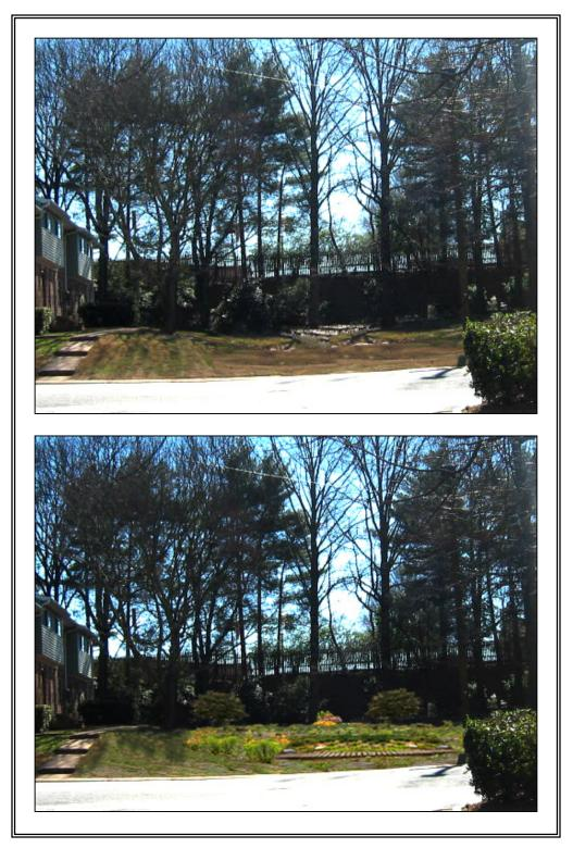
Figure 7.12 Frequently flooded from commercial parking lot runoff, before and after representation with rain garden installation
