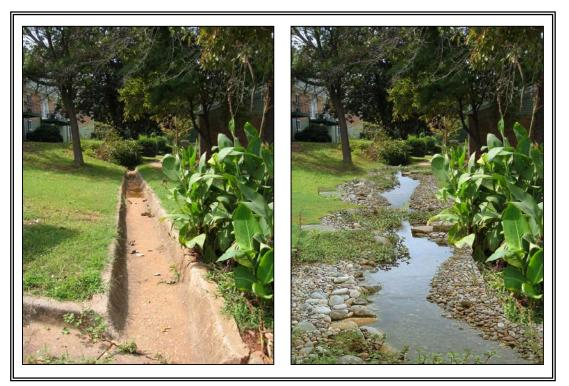
Figure 7.27 Vegetated courtyard, before and after—example of streambed installation
