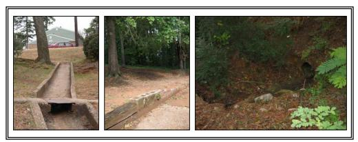
Figures 3.21 Fast moving runoff causes topsoil to be flushed away
