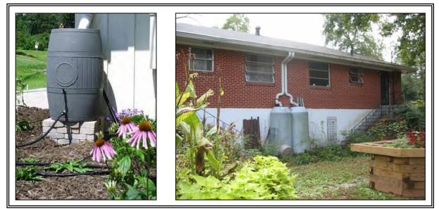
Figure 7.17 Examples of rain barrels to be used in the garden
