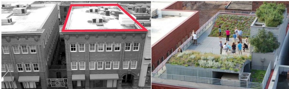
Figure 4.9 ASLA headquarters green roof before and after (Source: photograph by LAF, 2016)
