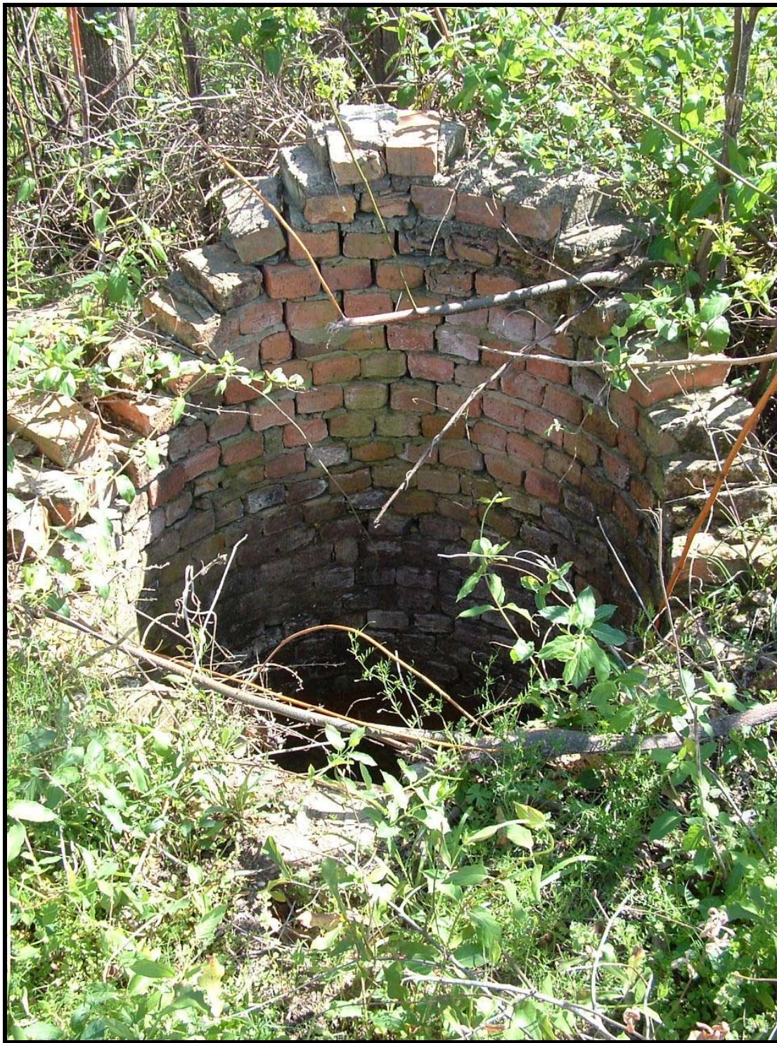
Forgotten Well Along Reid Road
