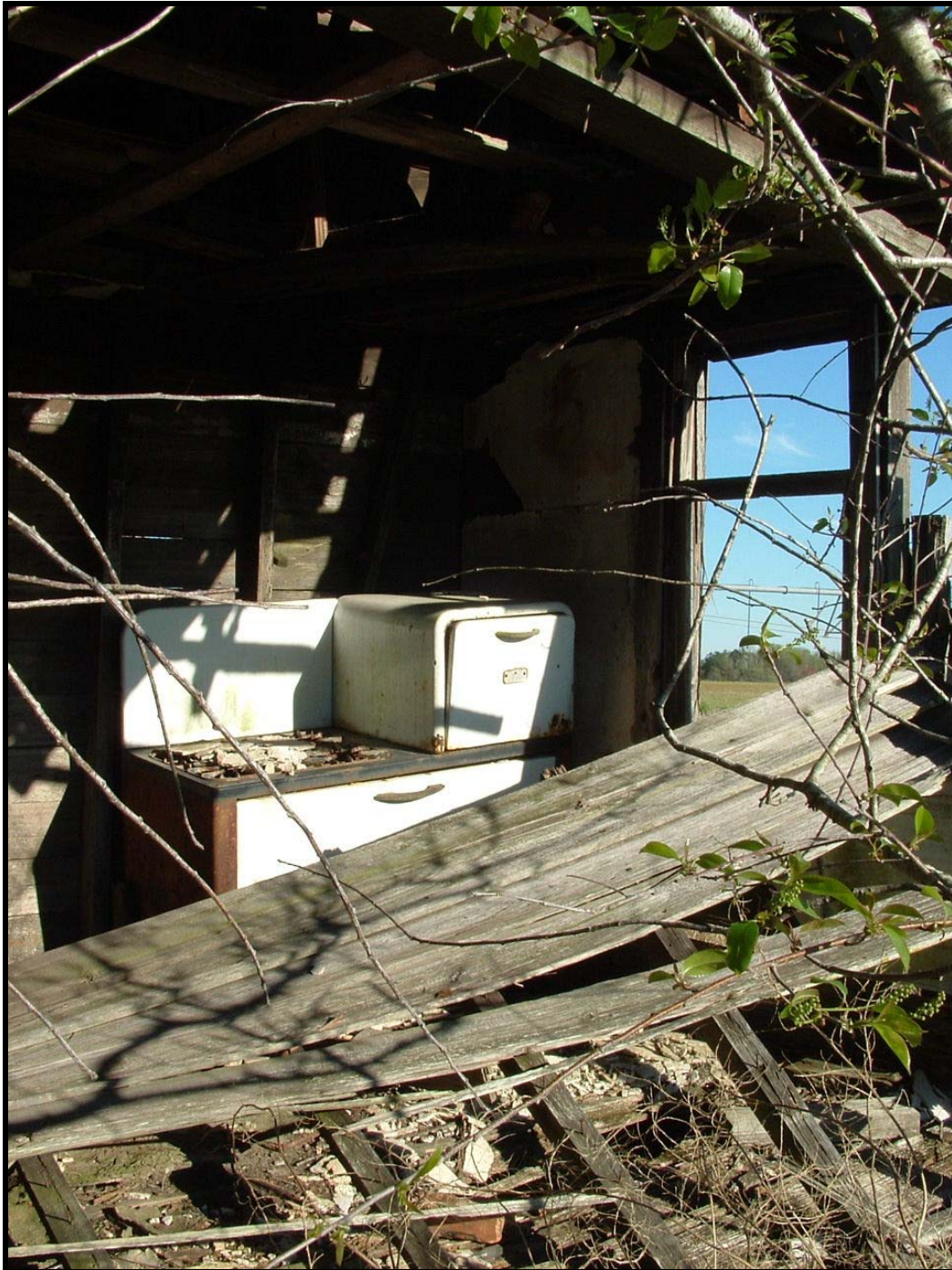
Demolition By Neglect Along John Pate Road
