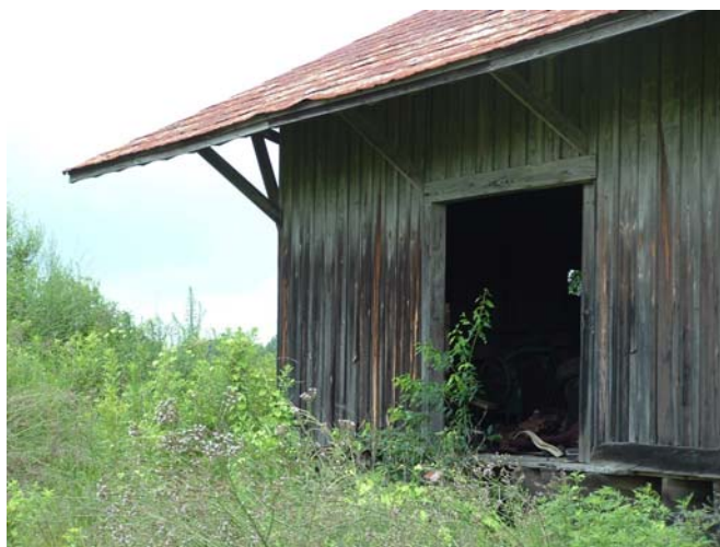
Figure 47: Turner County's Last Train Depot
