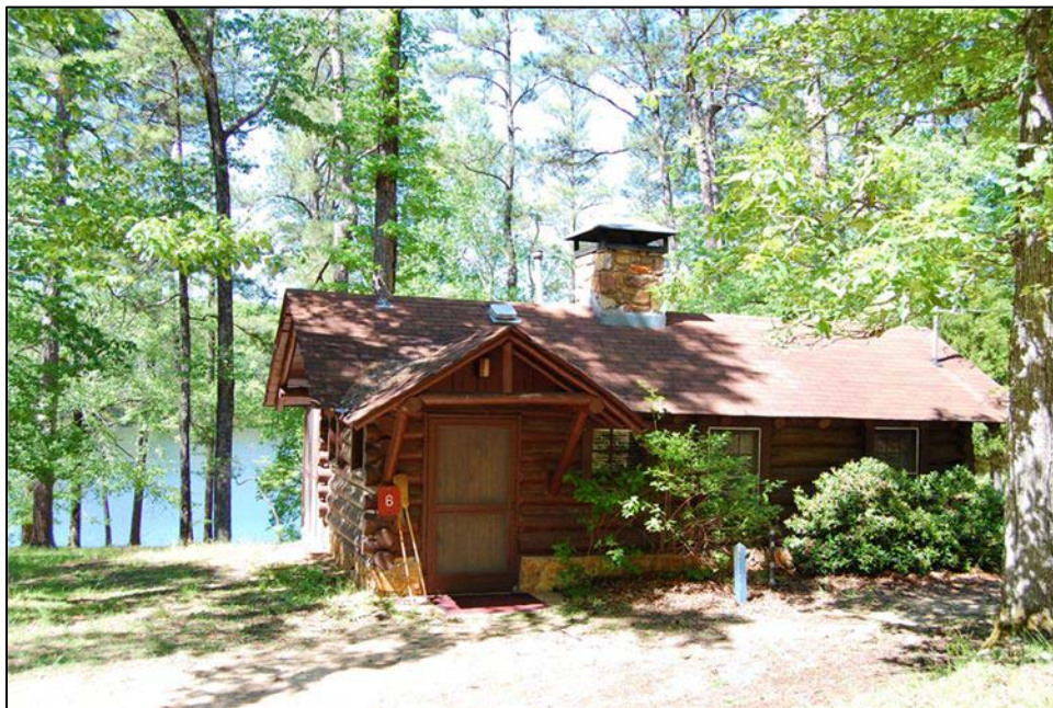
Figure 20: CCC-Constructed Cabin and Lake at FDR State Park. 133
