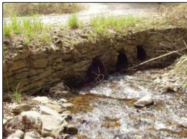
Figure 21: CCC-Built Culvert at Holly Creek. 143
