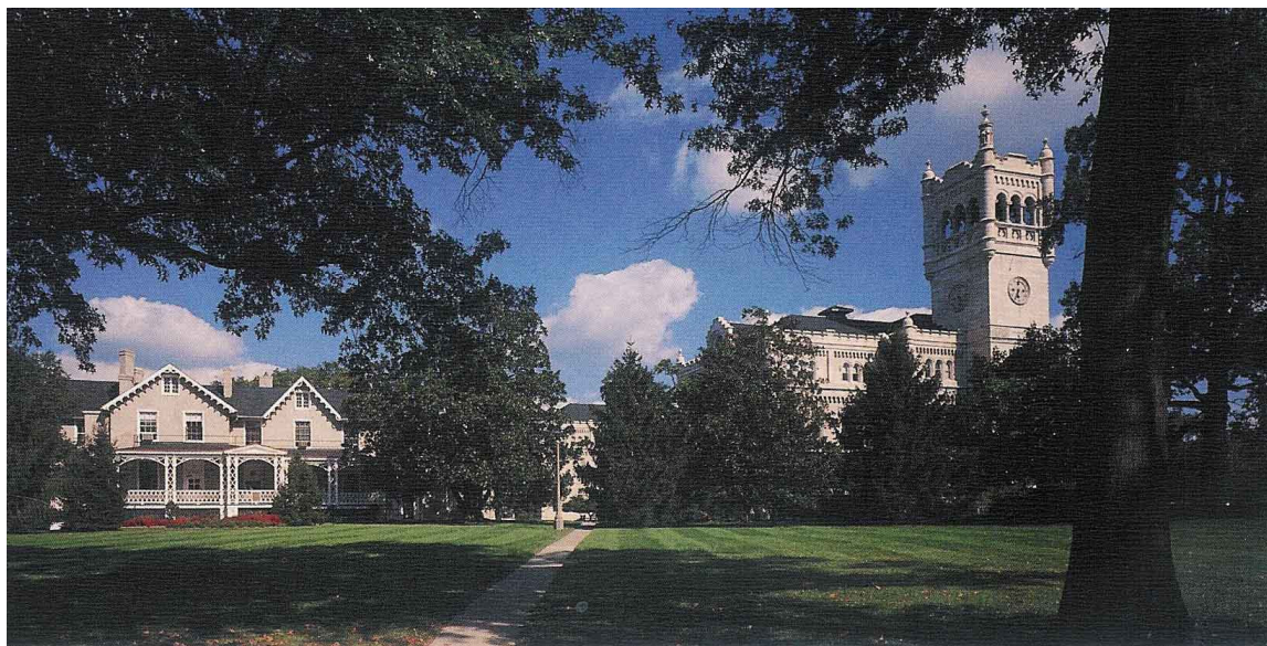
Figure 3.6 View of the south side of the property, Sherman Building on the right
