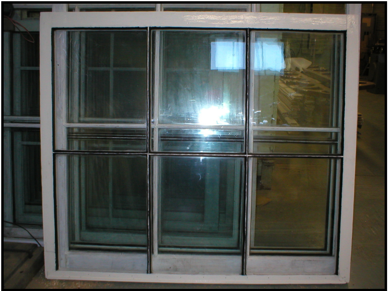
Figure 4.9 A stack of ‘almost’ restored windows - notice how the muntins almost disappear into the background when sun is shining on them
