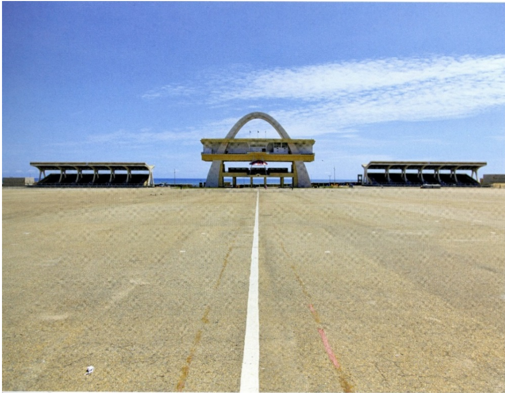
Figure 5.56: View of the Arch in Independence Square, Accra, Ghanaian Public Works Department (1961) 295
