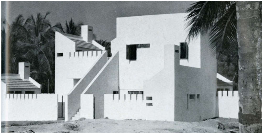
Figure 5.52: Housing Estate (1962), Christiansborg Castle (near Accra), D.A. Barrat. 286
