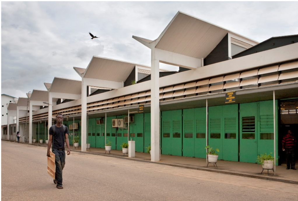
Figure 5.5: School of Engineering, KNUST, Kumasi (1956), James Cubitt & Partners. 158
