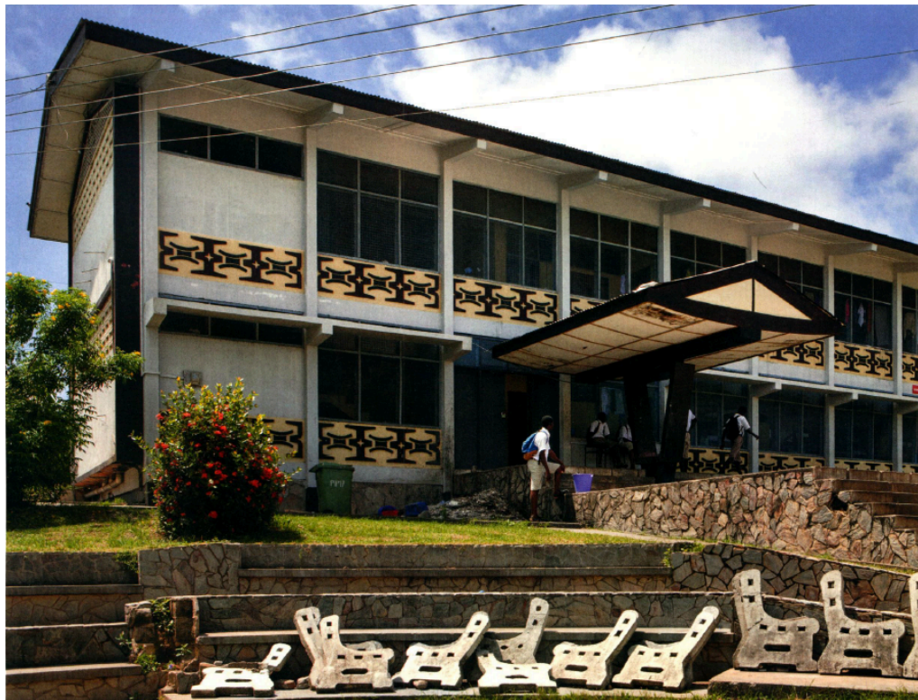
Figure 5.19: Exterior of Mfantsipim School, Cape Coast 189
