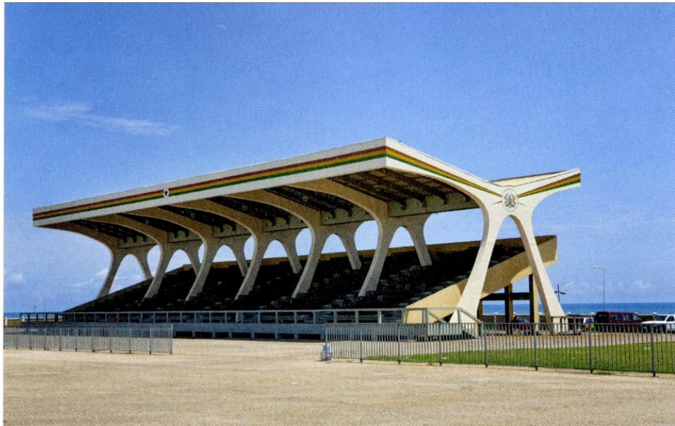
Figure 5.57: View of Ceremonial Grandstands in Independence Square. 296
