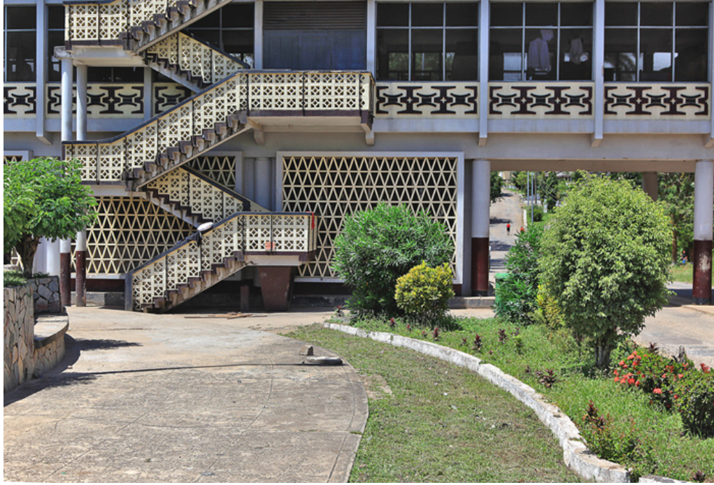
Figure 5.18: Exterior of Mfantsipim School (1958), Cape Coas, Fry, Drew & Partners. 188
