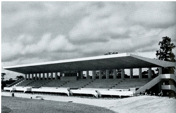
Figure 5.40: Kumasi Stadium, Kumasi, Grandstand, Kenneth Scott, c. 1960 256
