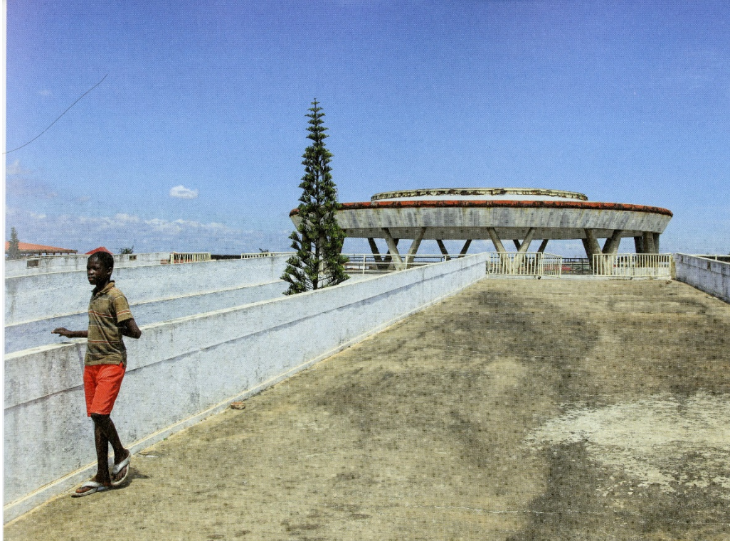
Figure 5.43: View of ramp to main entrance of the pavilion roof terrace, International Trade Fair 266
