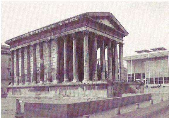
Figure 22 Maison Carrée (1 st century) and The Carré d'Art, Foster Associates, 1991. (Photo: The Architecture of Additions , 57)
