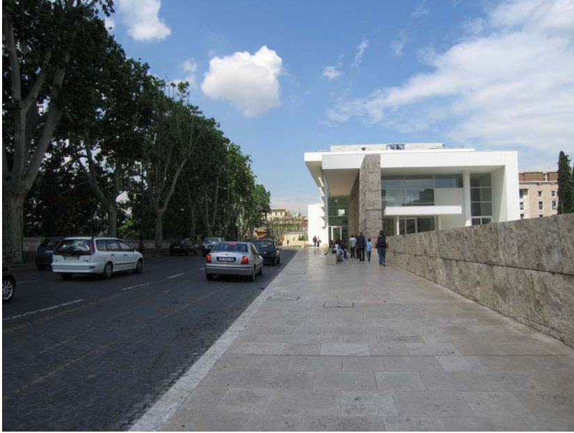
Figure 36 Ara Pacis Museum: front façade and travertine wall
