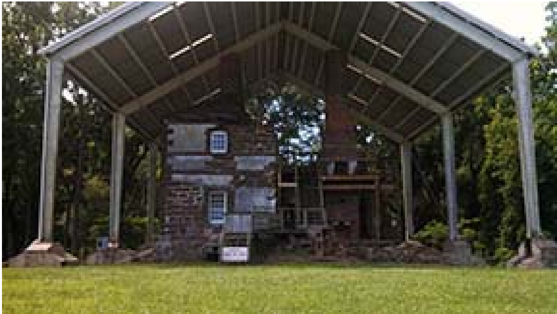
Figure 4.1 Menokin, photo taken by the author. A large metal superstructure protects the ruins of the mansion.
