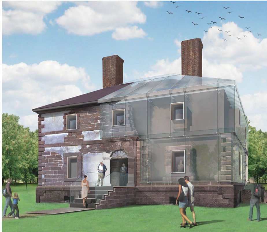
Figure 4.2 Machado and Silveti, Rendering of Menokin Glass House , found in “The Menokin Glass Project,” pg. 1. The missing elements of the feature will be recreated in glass
