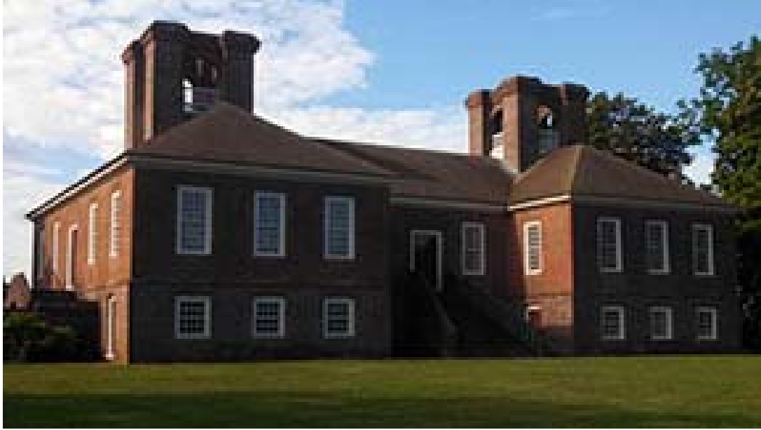
Figure 3.11 , The South façade of the Great House, Photo taken by author.
