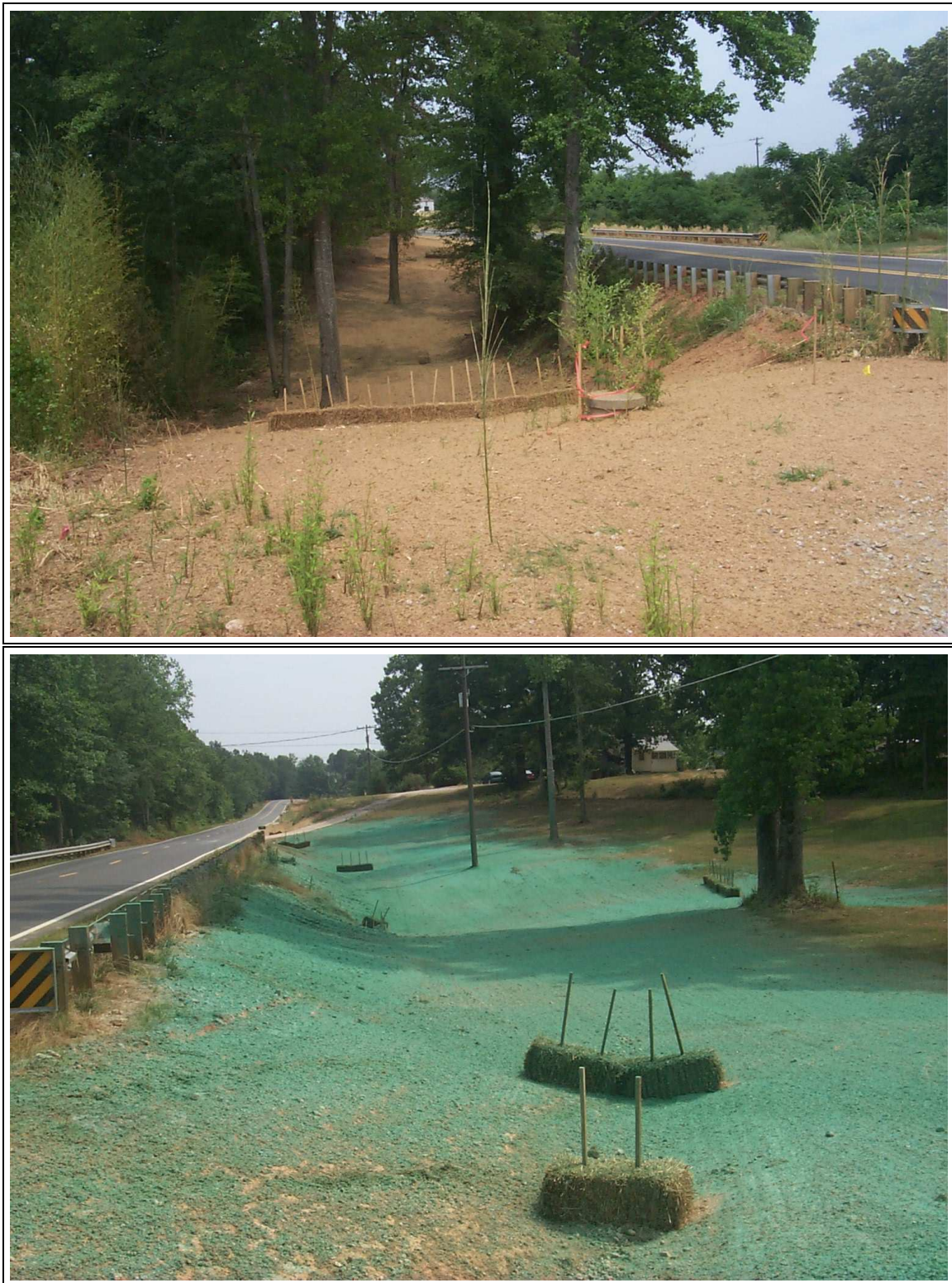
Figure 2.1: Examples of linear construction projects with Best Management Practices.
