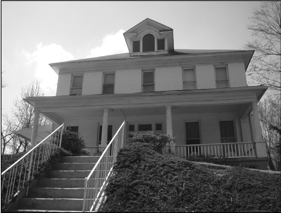
Figure 4.13. One of only a few larger historic structures that remain in Peoplestown
