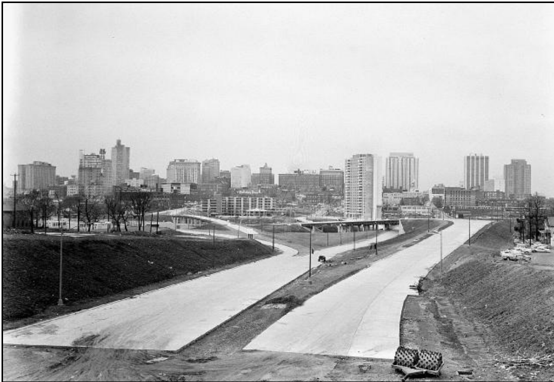
Figure 3.4. Highway construction in downtown Atlanta, early 1950s
