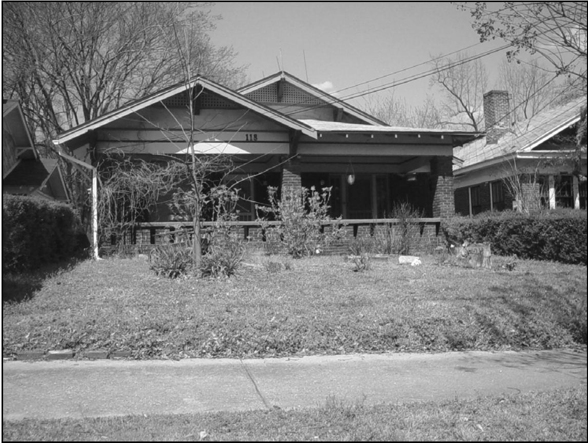
Figure 4.12. Historic house in Peoplestown
