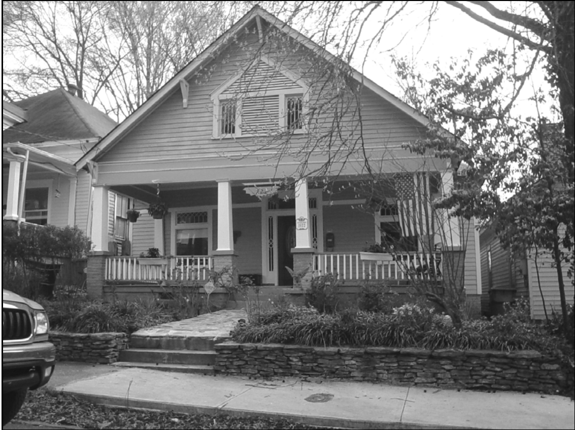
Figure 4.10. Historic house in Peoplestown
