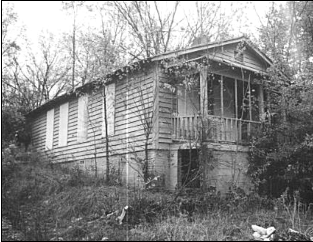
Figure 4.17. Deteriorating historic house in Peoplestown
