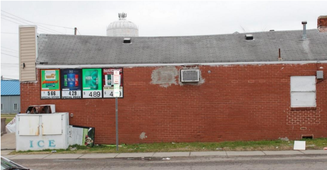
Figure 6.28 The East Elevation, along Peach Street, which shows the false front, rear chimney, and boarded window. Photo by Author.
