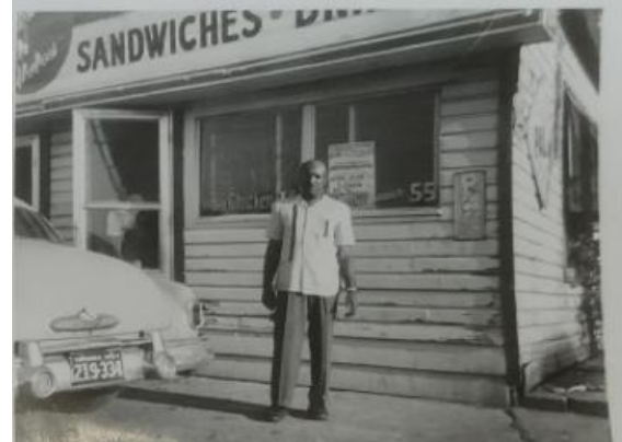
Figure 7.23 This photograph from 1954 also shows the wood siding, the historic window placement, and the original false front material.
