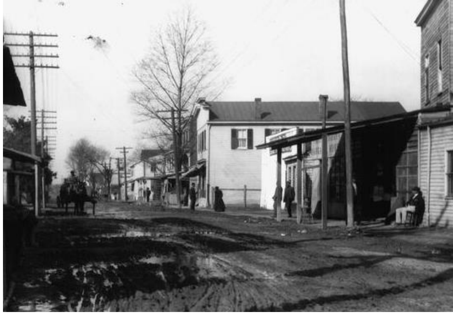
Figure 6.6 South Street Looking West from Chestnut Street, 1950s. While Watt's office would have been located behind the photographer, looking east from Chestnut Street, this photograph gives a feel for the neighborhood. Photo from the Portsmouth Public Library.
