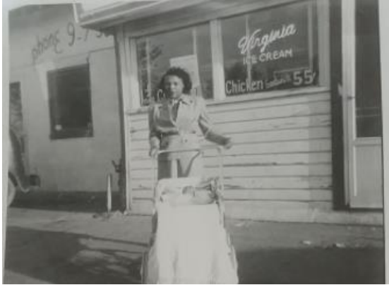
Figure 7.22 This photograph from 1954 shows the wood siding on Fagan's, as well as the historic window placement of the original building, and the now boarded over window on the expansion side. The material change of the false front can be seen here, contrasted with Figure 7.18.
