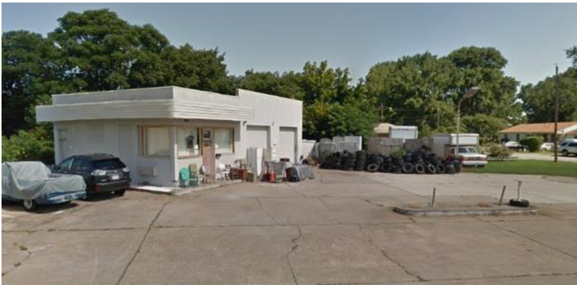
Figure 6.16 Marshall's Cities Service Station, East and South Elevation, 2017. The building features a curved decorative element around the top and a stepped roofline. Photo from Google Maps.
