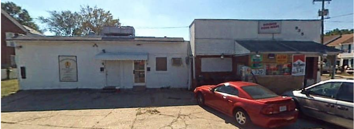
Figure 7.9 This 2007 photo shows the front addition on the original portion of Fagan's Restaurant. Google Maps.
