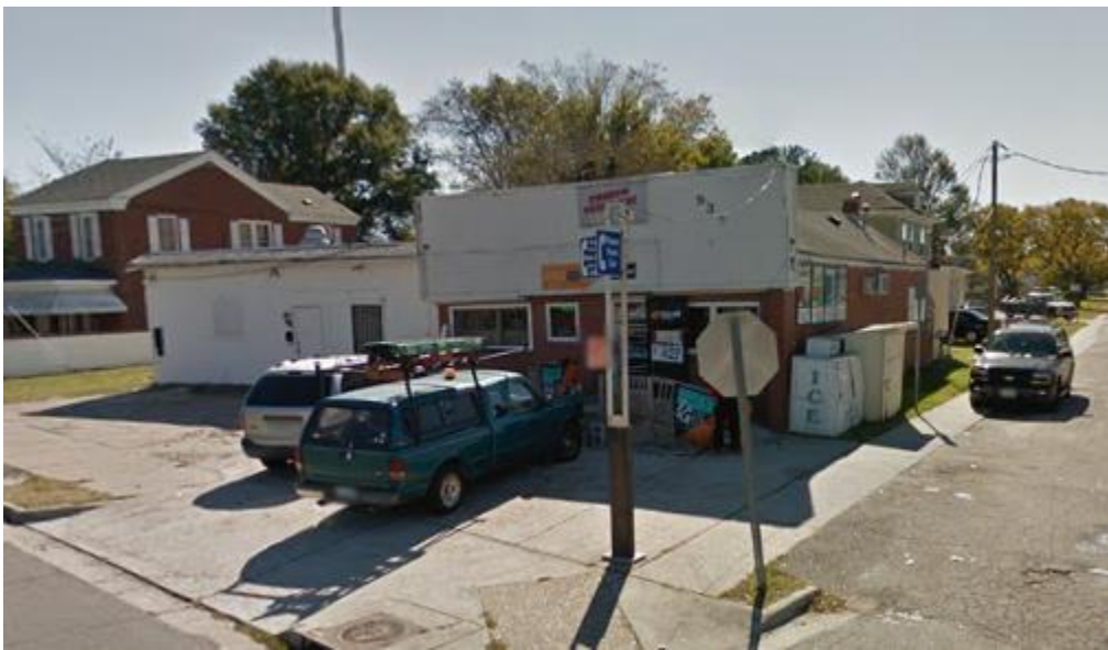
Figure 7.10 This 2015 photo shows the subsequent removal of the front addition. Google Maps.
