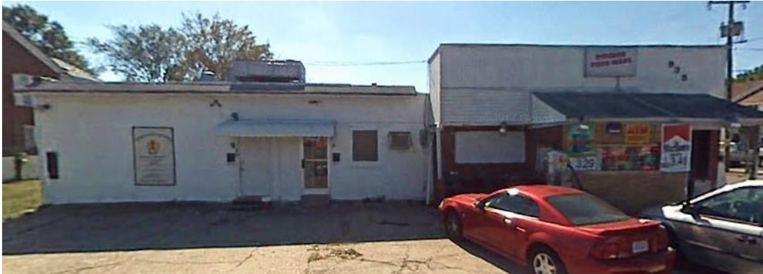
Figure 7.16 This 2007 photograph shows the boarded window and two single doors on the left side of the building, which Fagan's eventually expanded into. The original garage door on the left had already been removed. Google Maps.
