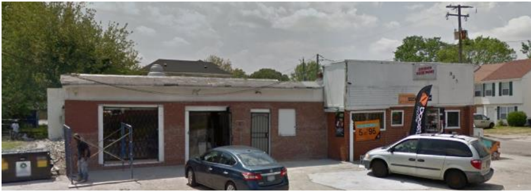
Figure 7.17 This 2016 photograph shows the major changes of the former auto repair shop, in the process of creating a larger door opening and a large fixed window. Google Maps.
