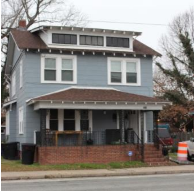
Figure 6.15 Raymond Durant's Residence at 3016 S. Elm Avenue, Front Façade East Elevation, 2017. There are clear Craftsman details, including the exposed rafter tails, the low-pitched roof, and the front porch. Photo by Author.
