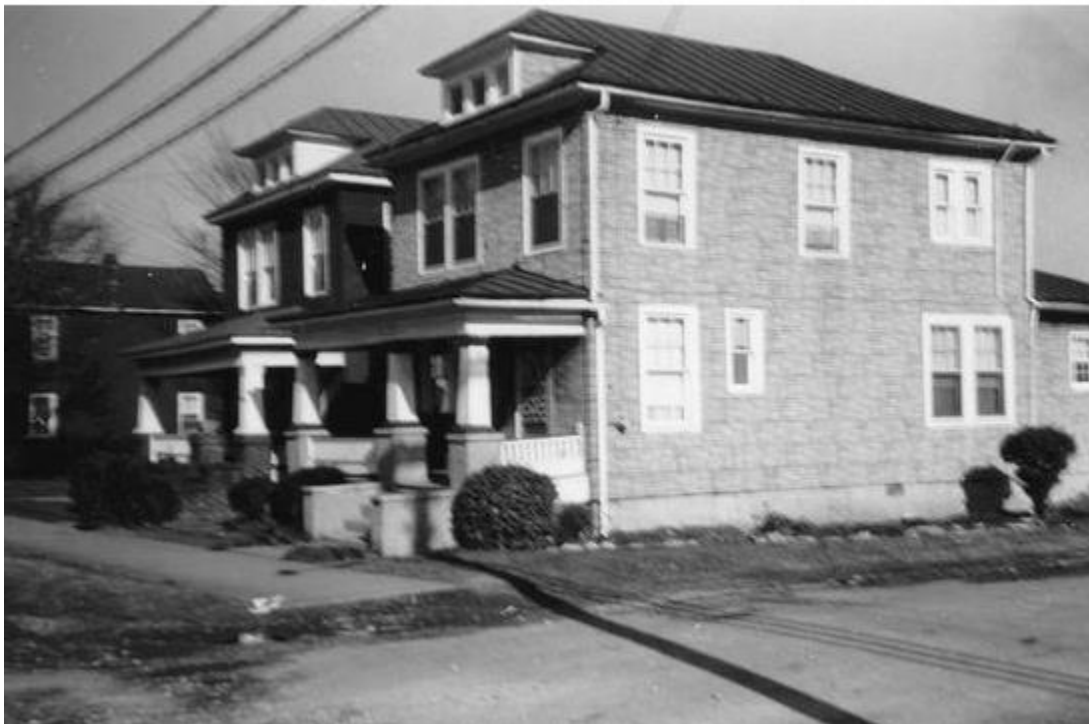
Figure 7.3 The historic photograph shows several buildings across the street from 3016 S. Elm, which give a hint to the historic character of the neighborhood. They are both still extant, adding to the historic setting and feeling of the area, while indicating what Durant's home may have looked like historically. Portsmouth Public Library.
