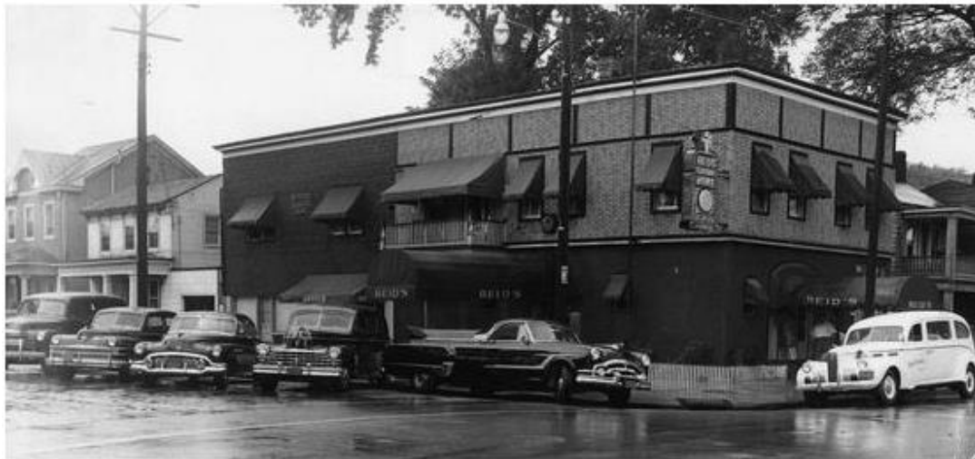
Figure 6.7 The Southwest corner of Effingham Street and South Street. Watt's office was located on South Street, west of Effingham. This photograph shows the area at a later date, after the roads had been paved. Photo from the Portsmouth Public Library.
