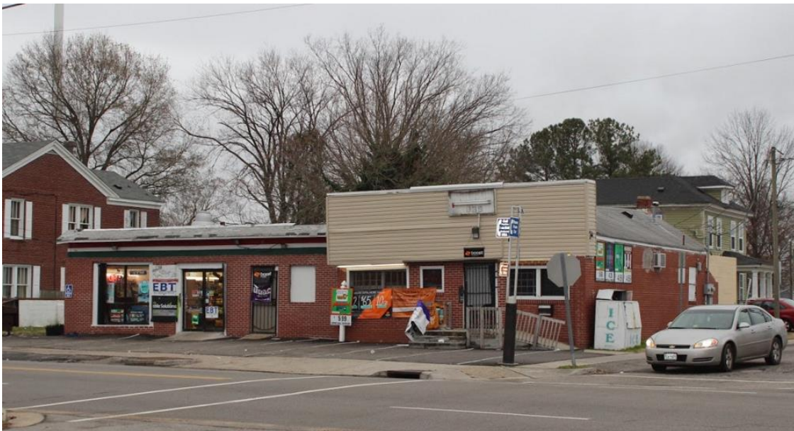
Figure 6.27 The front facade of 935 Portsmouth Boulevard, South Elevation, 2017. The storefront to the right, with the false front, is the original 1950s Fagan's Restaurant, while the portion to the left is where the restaurant expanded. Photo by Author.
