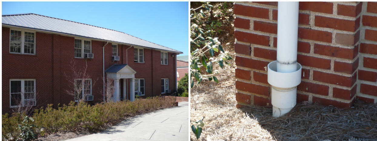
Figures 14 and 15: Military/ROTC Building: Built in 1941, the ROTC Building's (left) downspouts and gutters terminate underground (right) in a cistern (photos by S Stucker)
