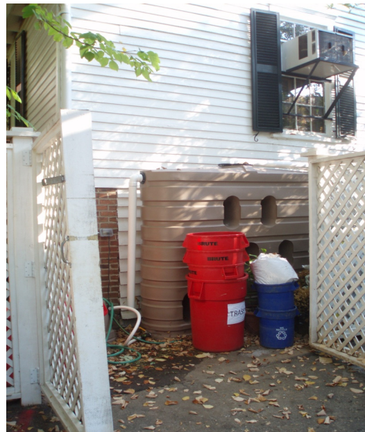
Figures 11 and 12: The Lumpkin House – Cistern: Water from the collector gutter passes through a filter (left), that removes leaves and other debris, before settling in the 540-gallon cistern (right) (photos by S Stucker/Kim Kooles)
