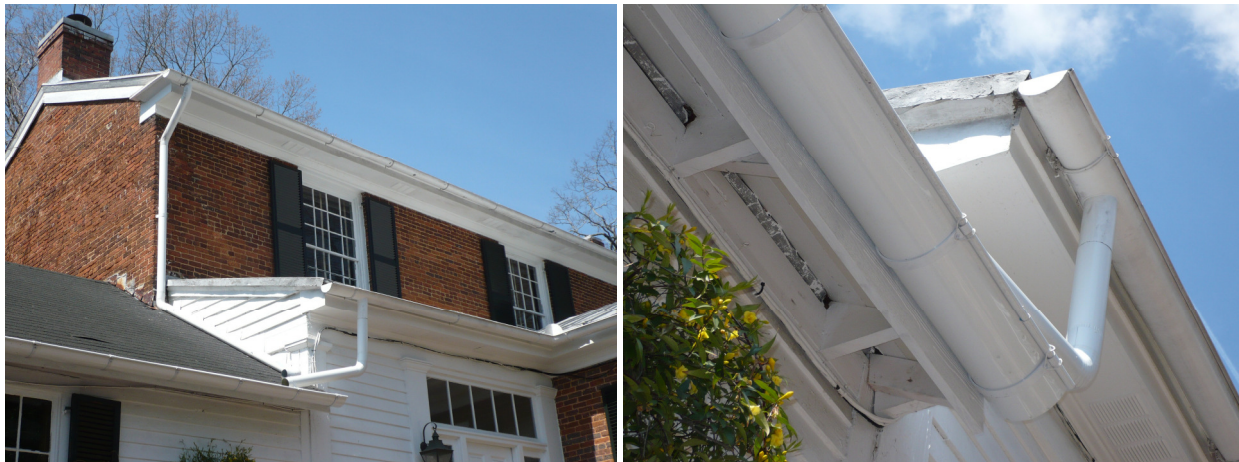
Figures 9 and 10: The Lumpkin House – Gutters and Downspouts: The gutters and downspouts for nearly half of the roof surfaces tie together (left), directing water into the larger collector gutter (right), which terminates in the cistern (photos by S Stucker)
