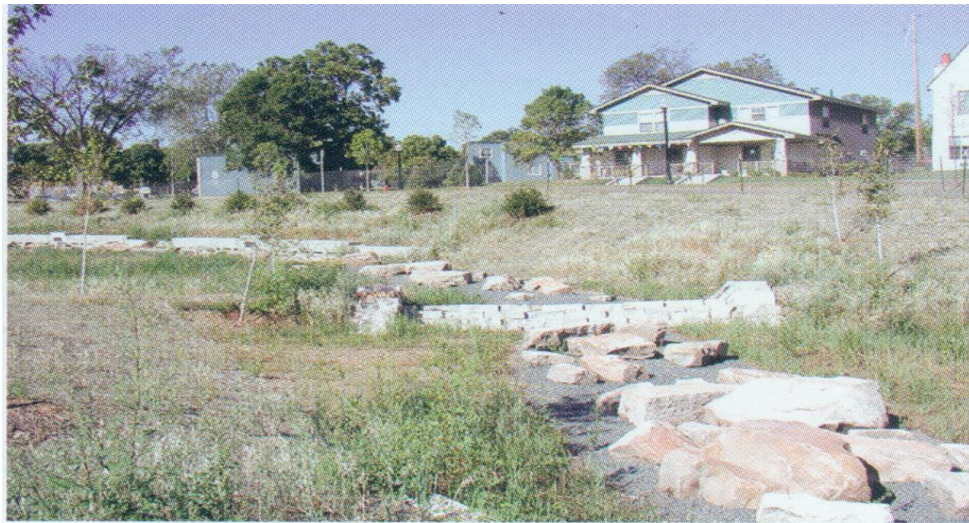
Figure 6: Bioswale: This bioswale is designed to look like a creek, adding both beauty and functionality to the landscape 129
