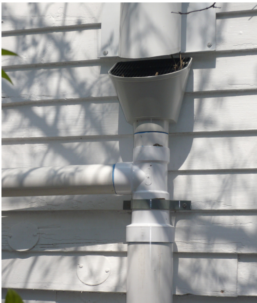
Figures 11 and 12: The Lumpkin House – Cistern: Water from the collector gutter passes through a filter (left), that removes leaves and other debris, before settling in the 540-gallon cistern (right) (photos by S Stucker/Kim Kooles)
