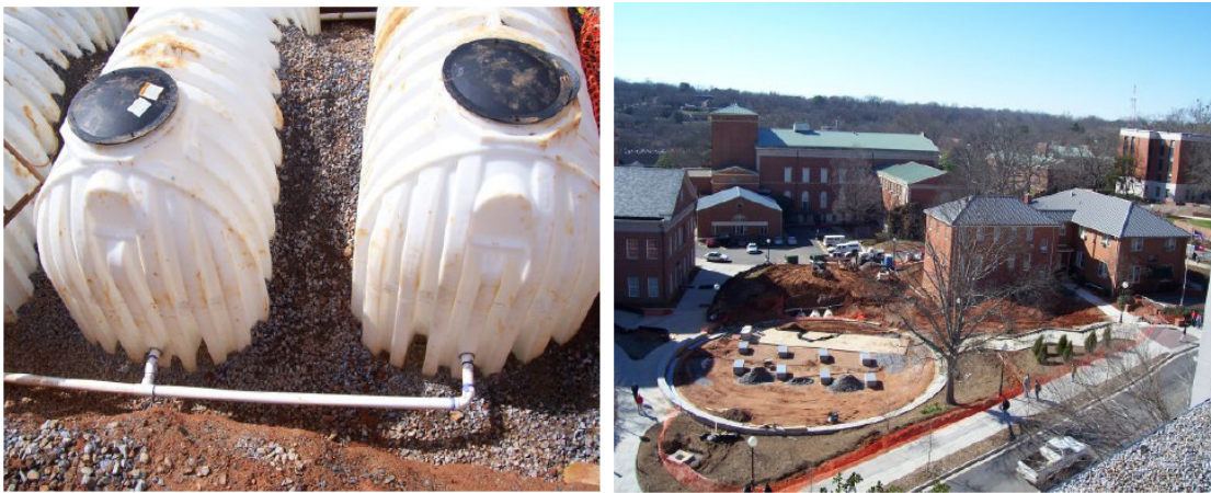
Figures 16 and 17: Military/ROTC Building – Cistern/Aerial View: Three 1700-gallon tanks linked together (left) are buried behind the ROTC building and are used to irrigate the Memorial Garden, shown under construction (right) 154
