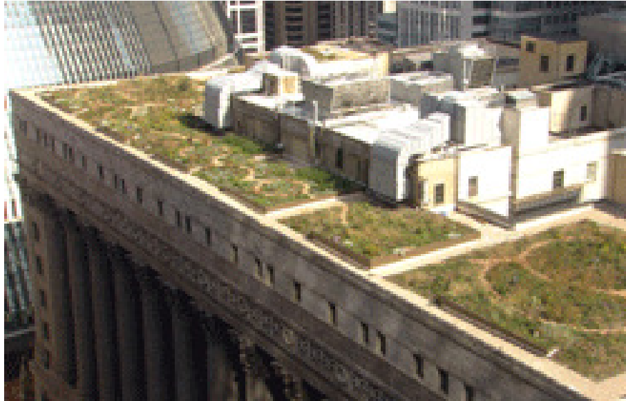
Figure 7: Chicago City Hall – Green Roof: The 20,000- square-foot green roof on Chicago’s City Hall “can retain 75% of a 1- inch rainfall before there is stormwater runoff into the sewers” 142
