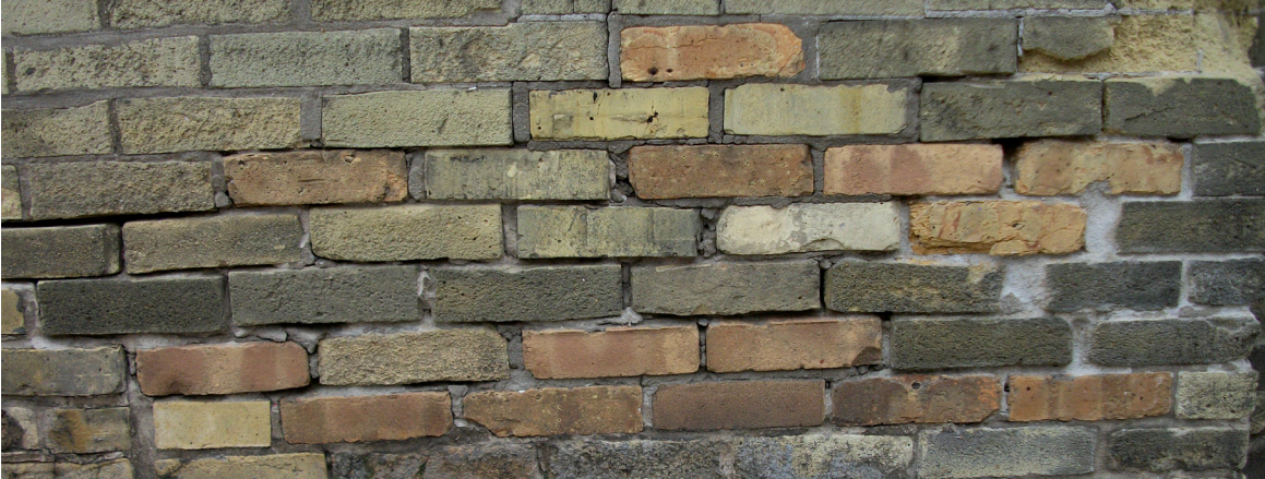
Figure 2.12: Wall showing various shades of Cream City brick in Milwaukee 99
