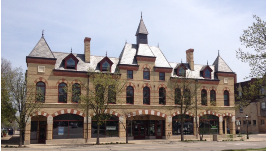
Figure 3.23: Arcade Building, Riverside, Illinois, following a 2010s restoration 216
