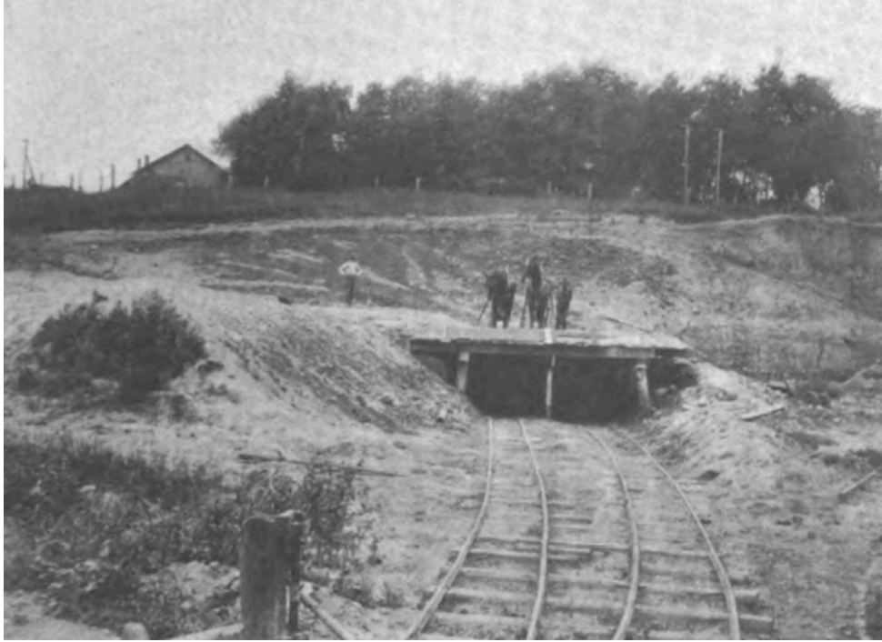
Figure 2.6: Clay pit of Davelaar & Son, Milwaukee, depicting mining method of plow and scrapers dumping clay onto a platform 68
