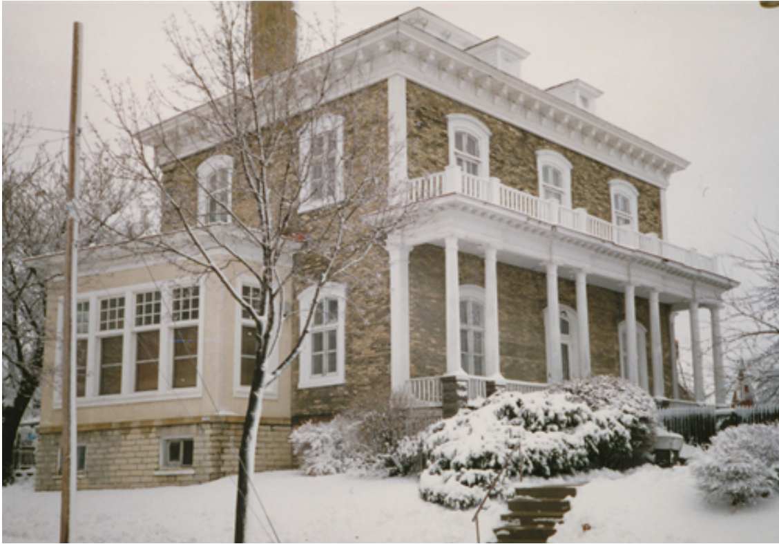
Figure 3.7: Villa Uhrig, with later side addition 183
