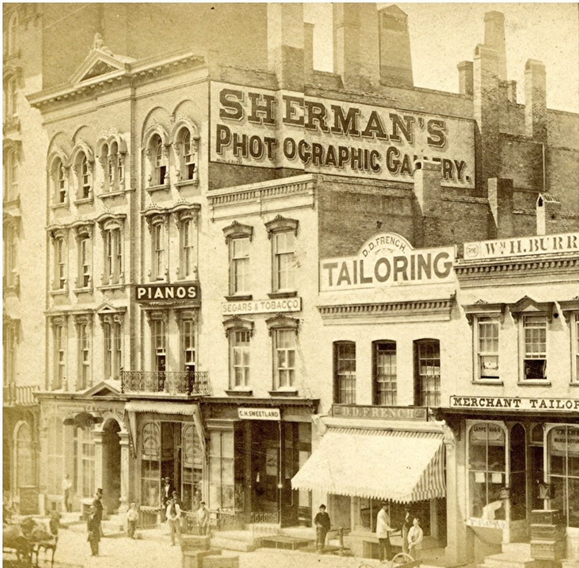
Figure 4.4: Downtown Milwaukee circa 1867 showing numerous Cream City brick commercial buildings 277
