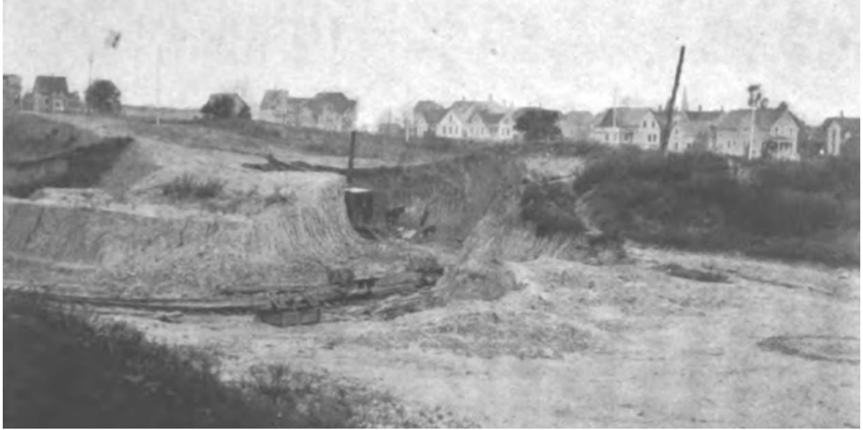
Figure 2.21: Clay pit of the Standard Brick Company 150
