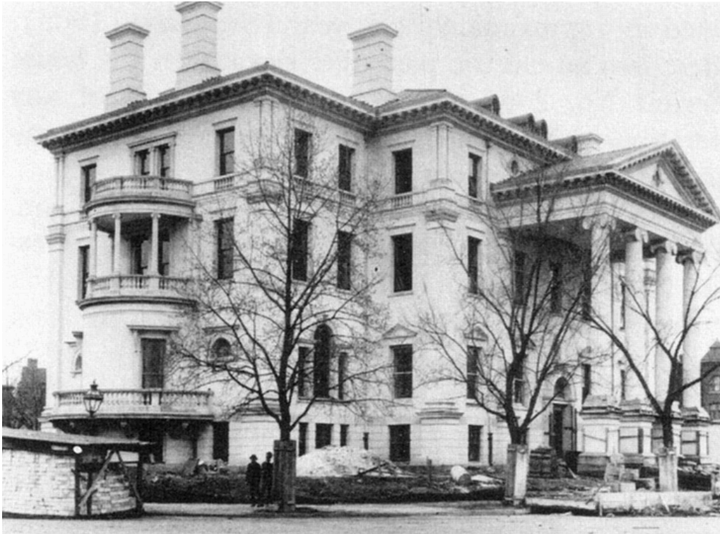
Figure 3.26: Levi Leiter Mansion during construction in 1893 230
