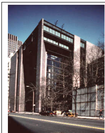
Figure 4.7: Planned patina, the Ford Foundation Building (1963-8, NYC), photo online: www.greatbuildings.com .
