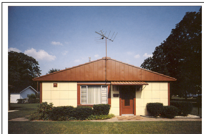
Figure 3.8: Lustron house number 2329, (1950, Chesterton, IN). (Reprinted from Thomas Jester, Twentieth Century Building Materials , 31. © 1995 by: McGraw-Hill.)
