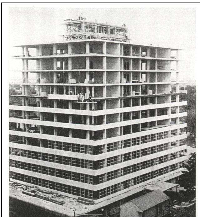
Figure 8.4: Construction of Drayton Arms, showing reinforced concrete, cantilevered design surrounding a central core. (Reprinted from “Apartment House Construction Methods.” Progressive Architecture 33, no. 11, 83. © 1952.)
