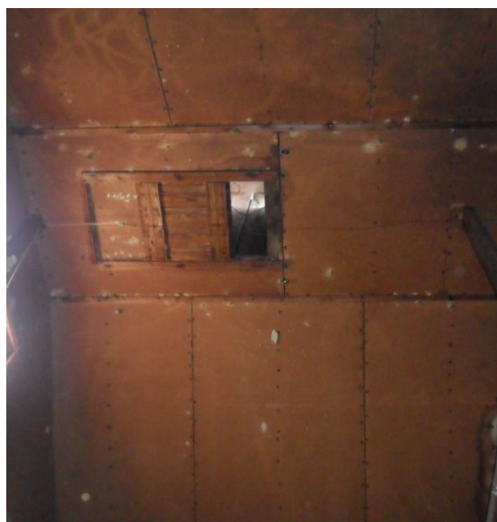
Figure 3.15: Insulation on the Ceiling
