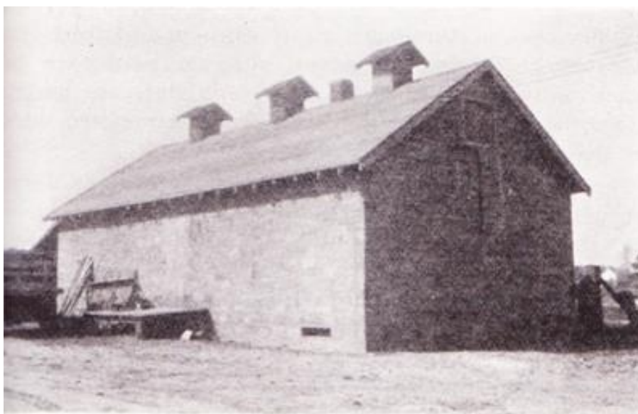
Figure 3.5: Concrete Block Sweet Potato Curing Barn - Princess Anne County, Virginia 57
