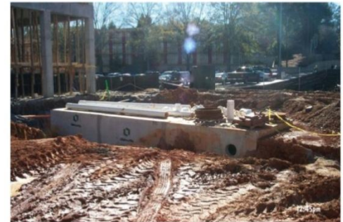
Below: Cisterns during installation at Coverdell.
