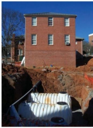
Left: Cisterns during installation at Memorial Garden.
