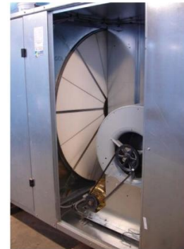
Fig 2-3: Energy Efficient Mechanical System using Heat Wheels
