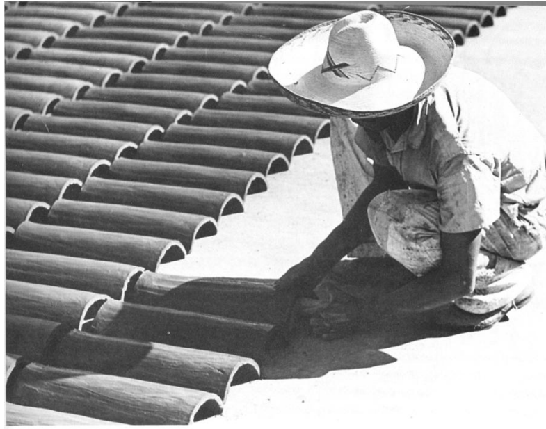
Figure 4-1: Placing the red clay roofing tiles, which were created on site using kilns
