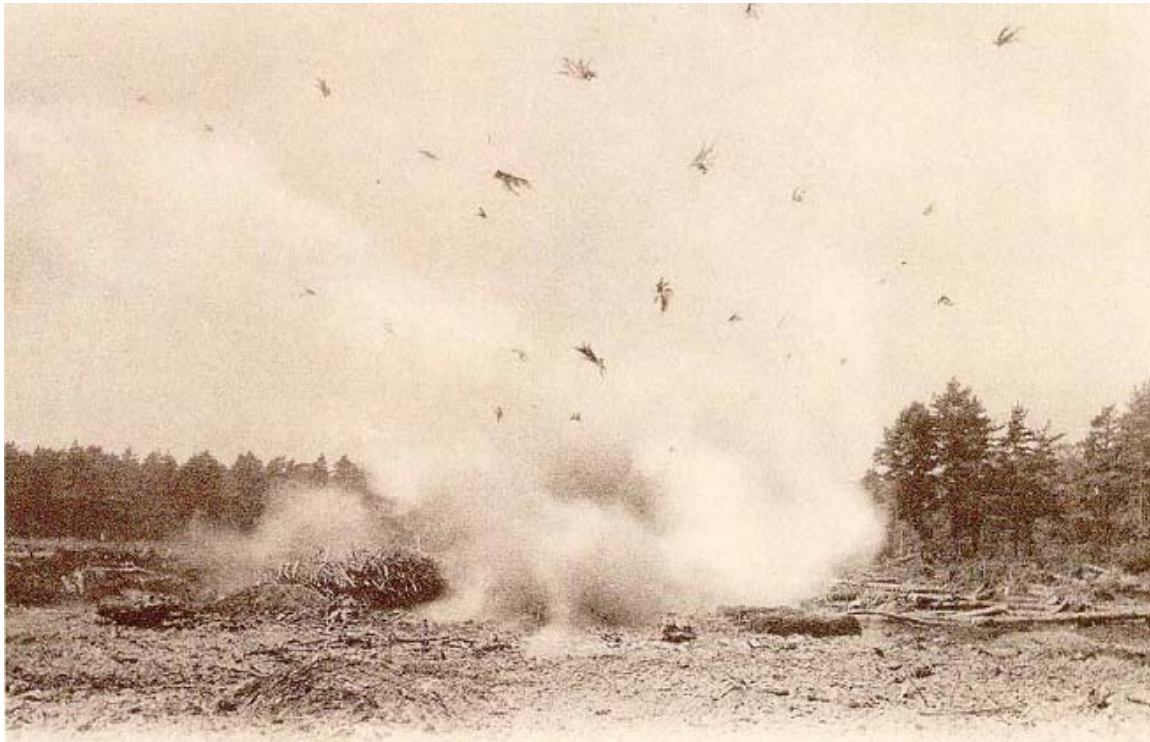
Figure 3.5: Dynamite was used to clear dense forests.
