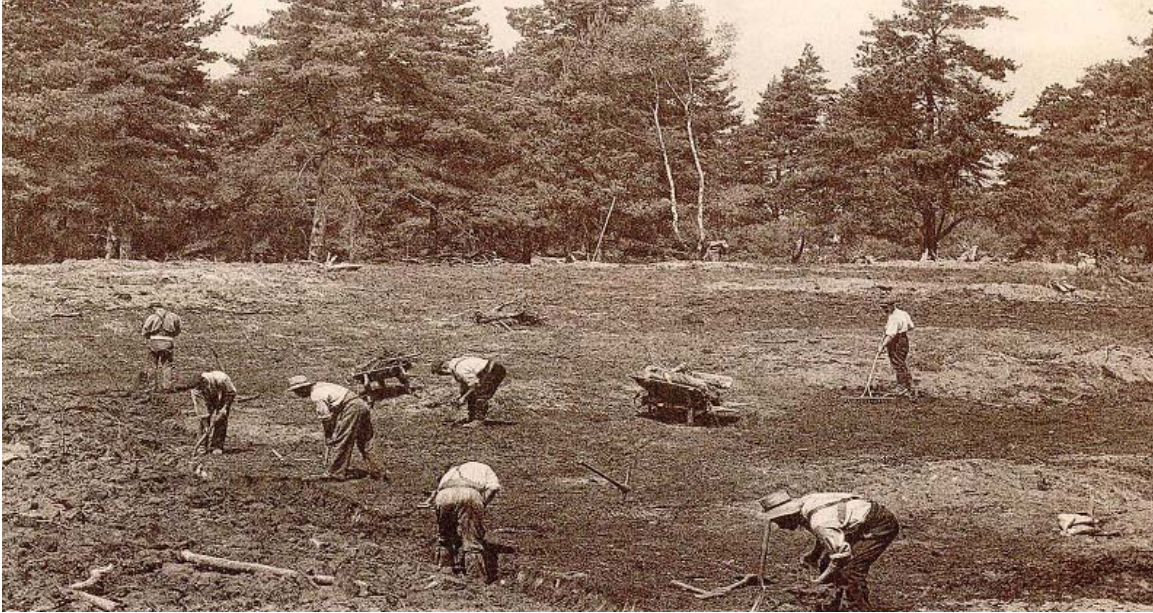
Figure 3.6: Large amounts of manual labor was also needed to help clear the land.
