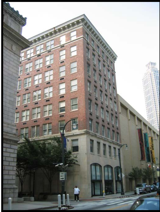
Figure 15- Haas Howell Building front and side facades
