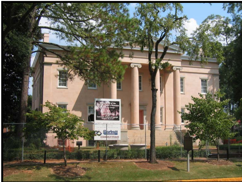
Figure 30- Current restoration efforts on the Old Governor's Mansion.
