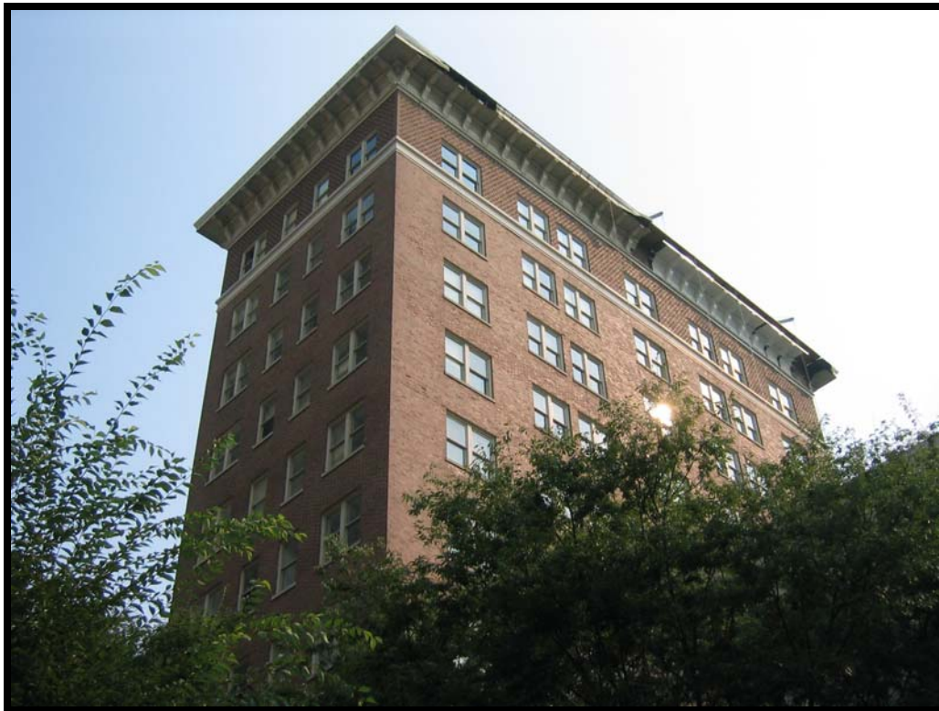
Illustration 18- Standard Building, front and side facades
