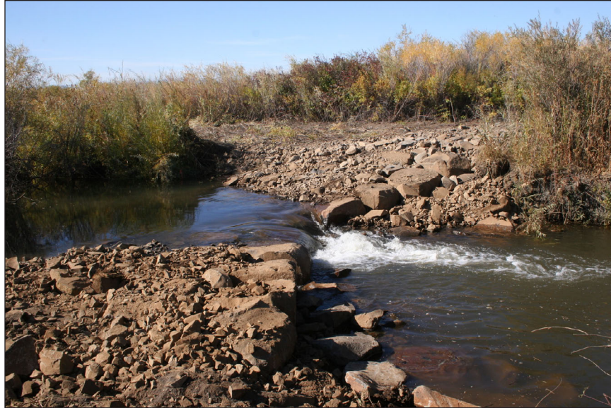
Figure 29. Grade control structure on Toppenish Creek. This lifts the water level, flooding dewatered historic channels and decreasing erosion, while allowing anadromous fish passage.
