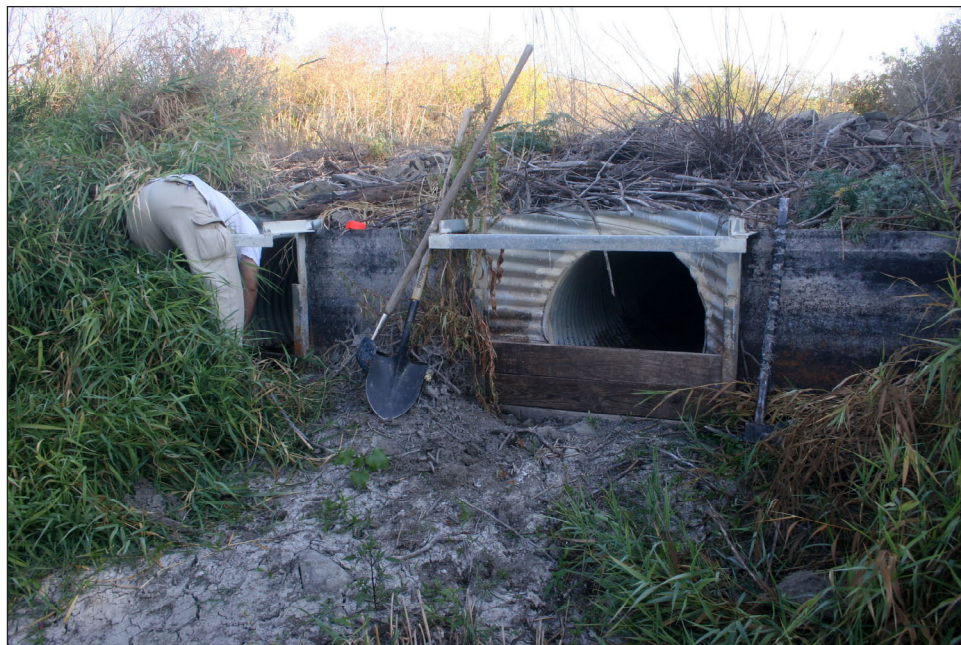
Figure 22. Culverts with flashboard risers. Boards can be stacked or removed to raise or lower the water level in the impoundment.
