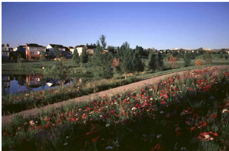
Figure 3.12 Detention pond near a Housing Complex, Colorado (Urban Drainage Criteria Manual, 2001, DP-11)
