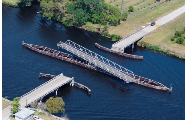
Figure 2.4. Okeechobee Waterway, Florida Swing Bridge
