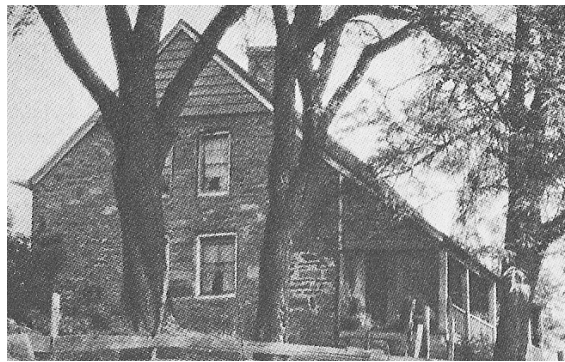
Figure 4.34: Evert Terwilliger House, Plattekill, New Paltz, after 1760s modernization; the original entrance was on the gable end, but it was relocated to the right side when modernized.
