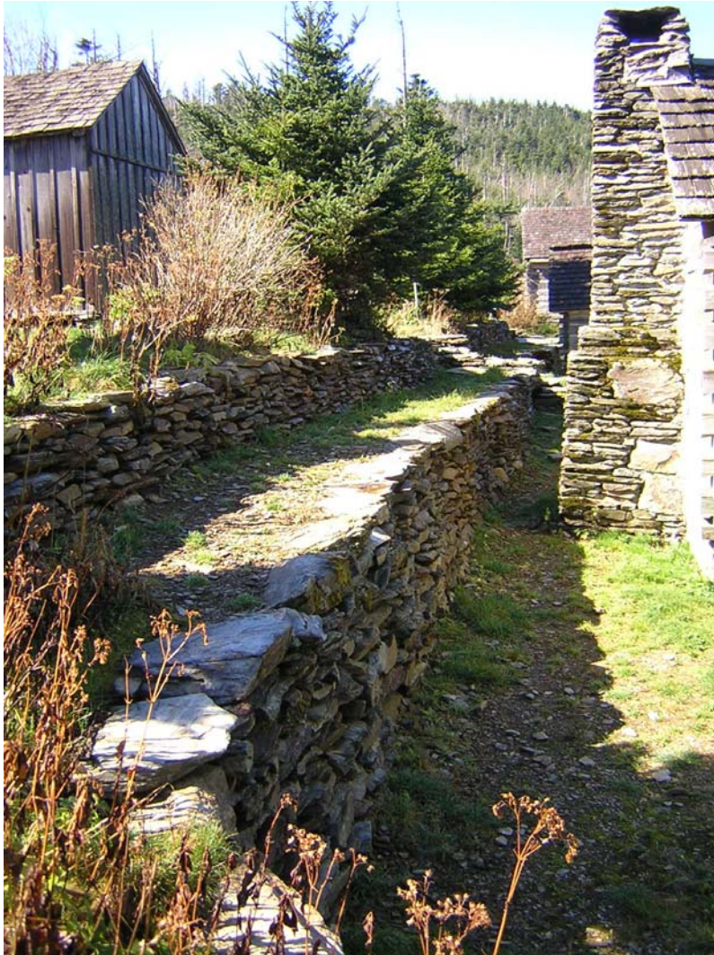
Figure 3.15 Reconstructed walls behind the New Lodge. October 24, 2004 Photographer: William Shealy (author)
