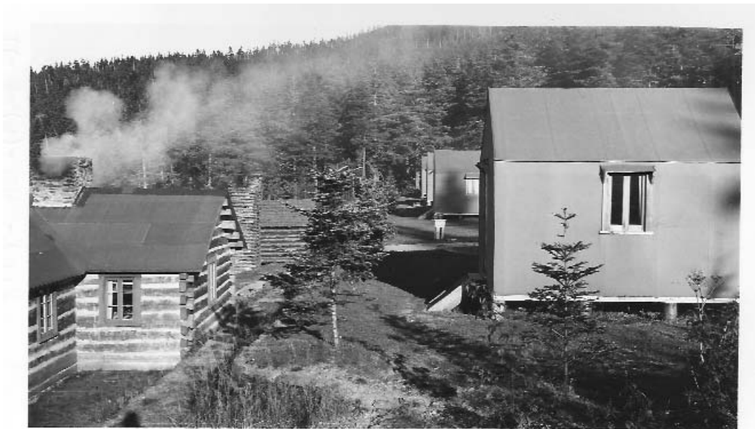
Figure 2.4 Cabins with asphalt paper walls and roof. 1947 Photograph courtesy of the Great Smoky Mountains Library
