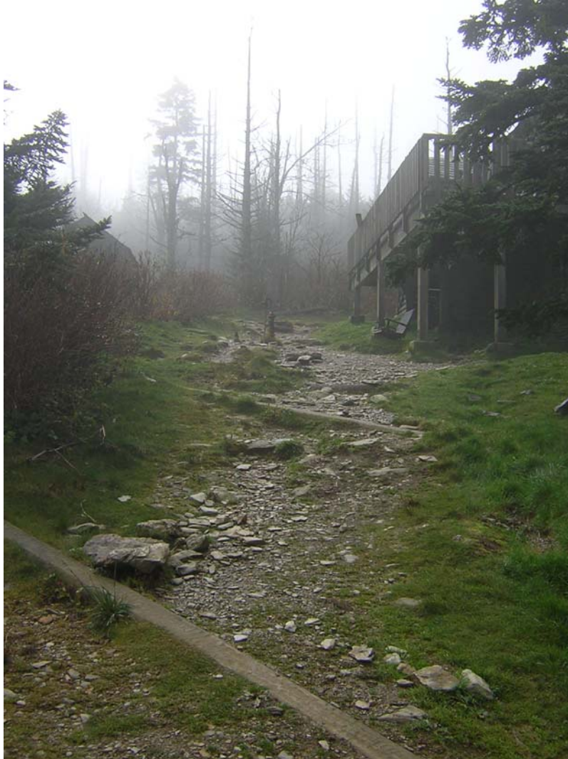
Figure6.6 Erosion along path between Cabin Four and woodshed. October 24, 2004 Photographer: William Shealy (author)
