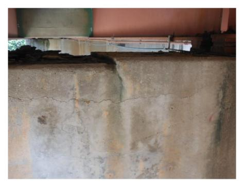
Figure 16—Horizontal Crack in Bent Cap [GDOT, 2017]
