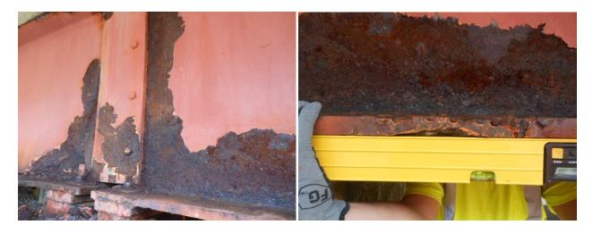
Figure 15—Superstructure Deterioration: (a) Deterioration in Web and Bottom Flange (b) Section Loss of 0.25 in [GDOT, 2017]
