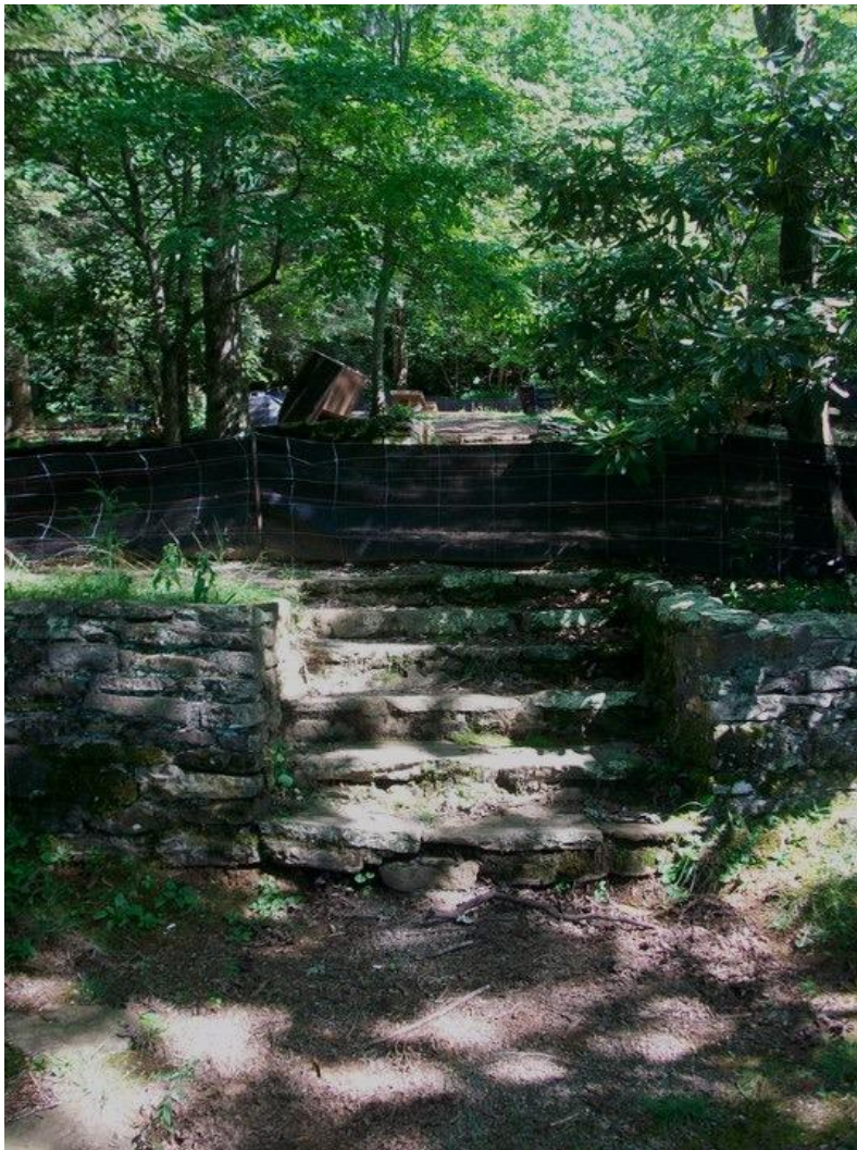
Figure 4.3. Stairs leading from the second terrace to the picnic area and further toward the third and final terraced section beyond the erosion screen, 2009. (Photo source, Darby Phillips Miller.)
