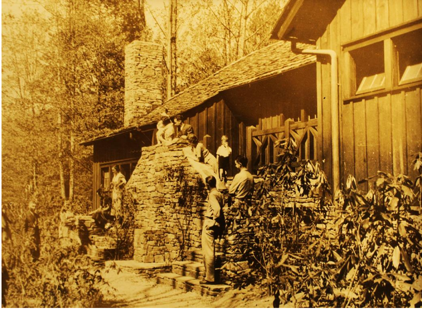
Figure 3.6. West elevation of the CCC-era bathhouse constructed circa 1936. Notice the wall of windows in the center of the photo which was removed in between 1950 and 1955. The men's section is located to the north (left side of building), with the women's to the right. (Photo source, U.S. Forest Service, Blue Ridge Ranger District Office, circa 1950.)
