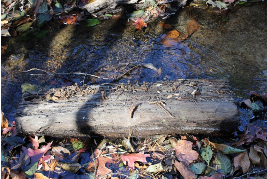
Figure 4.11. Foot bridge timber, hand hewn with wire-cut nails where planks were attached. (Photo by M. Scales English.)
