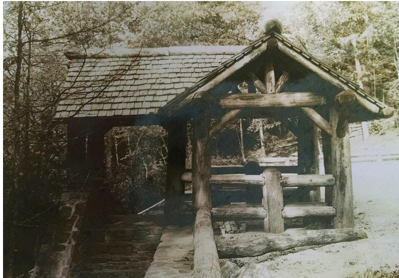
Figure 3.5. Original fee-booth structure located on the western side of the main parking lot and at the top of the stairs leading to the bathhouse. Wood shingles and rounded timbers were harvested on-site. (Photo source, Blue Ridge Ranger District Office, Blairsville, Georgia.)
