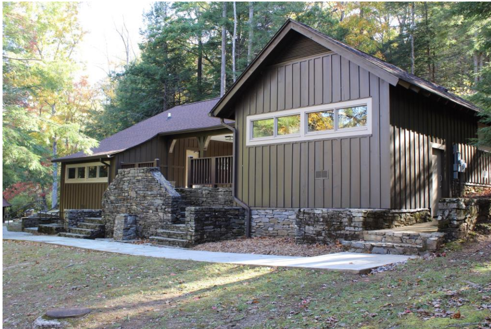
Figure 4.4. CCC-era bathhouse, existing conditions (2016); retention of the board-and-batten siding and stone foundation adds to the integrity of this resource. Despite changes to the breezeway and entrances, this building has been rehabilitated to maintain similar appearance of the original configuration. (Photo source, M. Scales English.)
