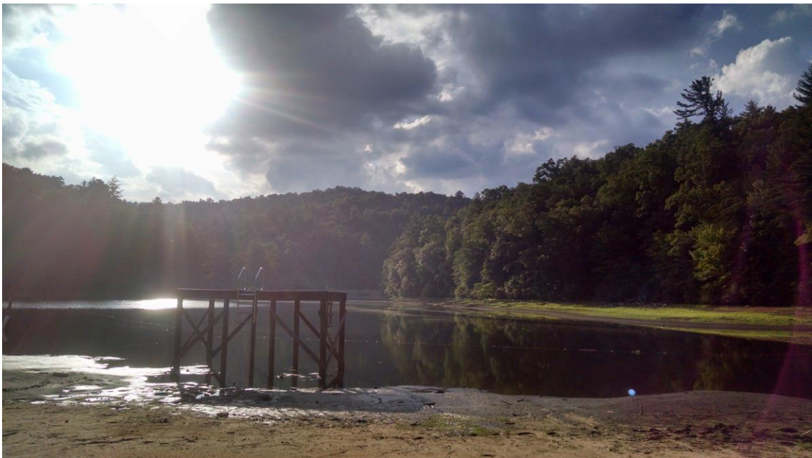
Figure 5.1. This image illustrates the dramatic drop in water depth due to the faulty drain pipe at Lake Winfield Scott. The height of this platform dock is roughly ten feet. (Photo source, M. Scales English, August 2016.)
