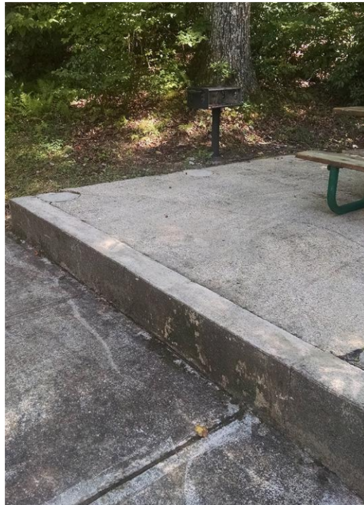
Figure 3.11. Remnant of the Shelter 2 concrete platform remains. Notice the timber post mold's shape (upper right-hand corner) is circular at this shelter (2016). (Photo source, M. Scales English.)
