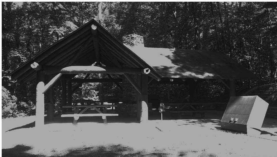
Figure 4.5. Shelter 1, south elevation (2016) . (Photo by M. Scales English.)
