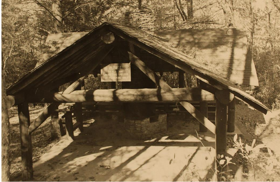
Figure 3.7. East elevation of day-use Shelter 1 (circa 1935); notice the round timbers compared to the squared timbers of Shelter 3 in Figure 3.9. (Photo source, Blue Ridge Ranger District, Blairsville, Georgia.)
