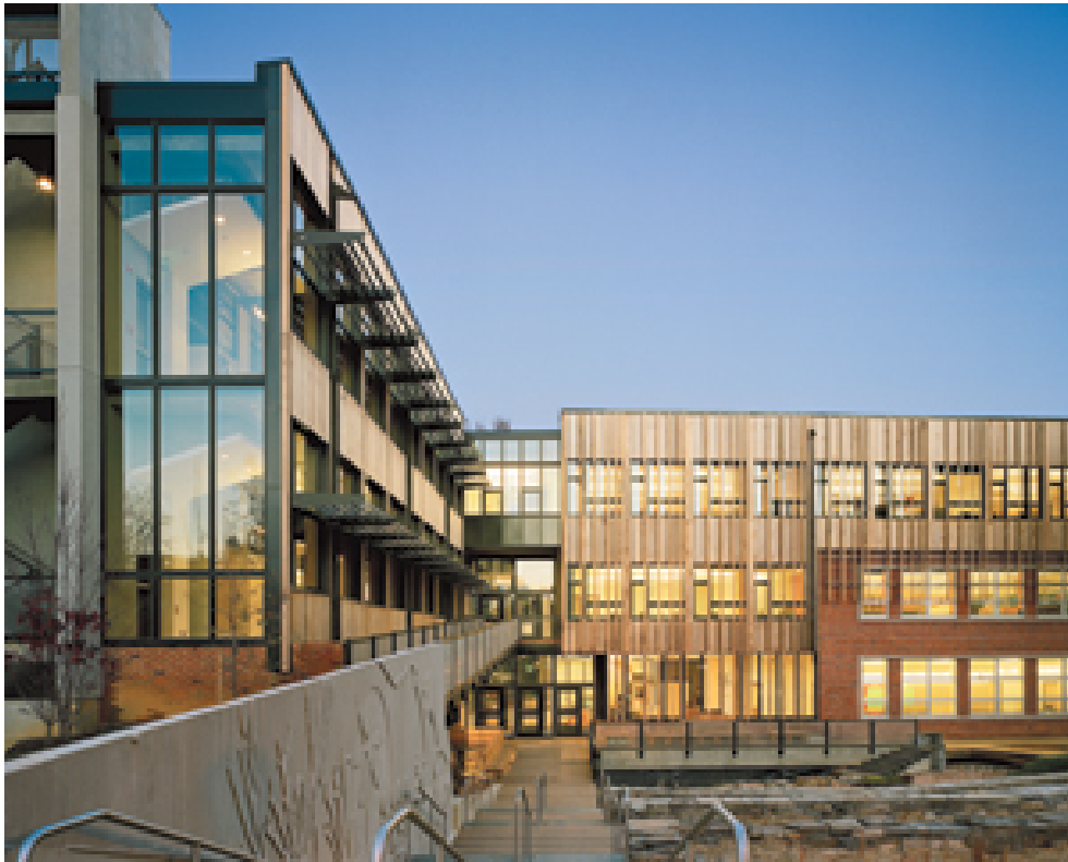
Figure 23. Recycled wine barrel cladding (Associates)
