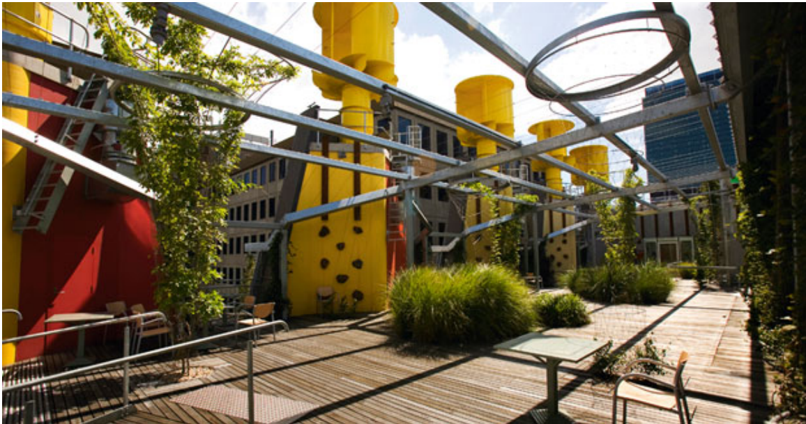
Figure 17. Water Capture System along CH 2 Roof (Antony Wood 2014)
