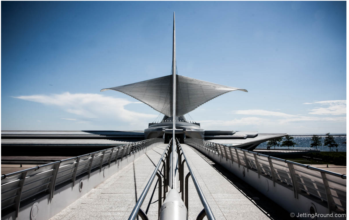
Figure 13. Burke Brise Soleil, Extended (Henderson 2013)
