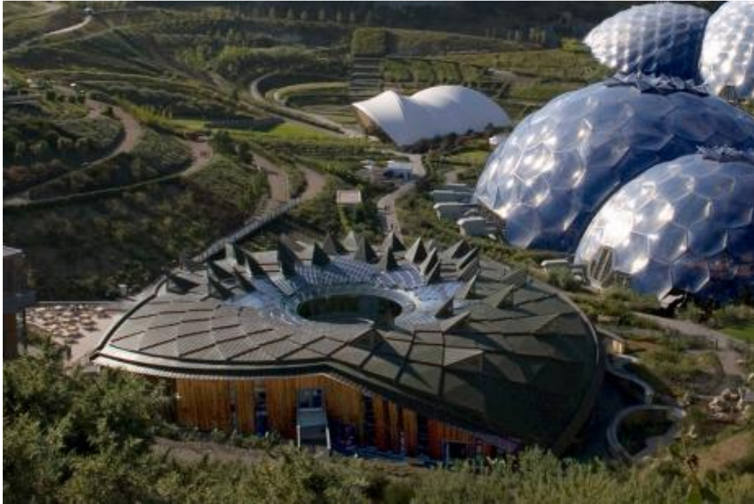
Figure 10. Trunk and Canopy Roof of the Core (Architects)
