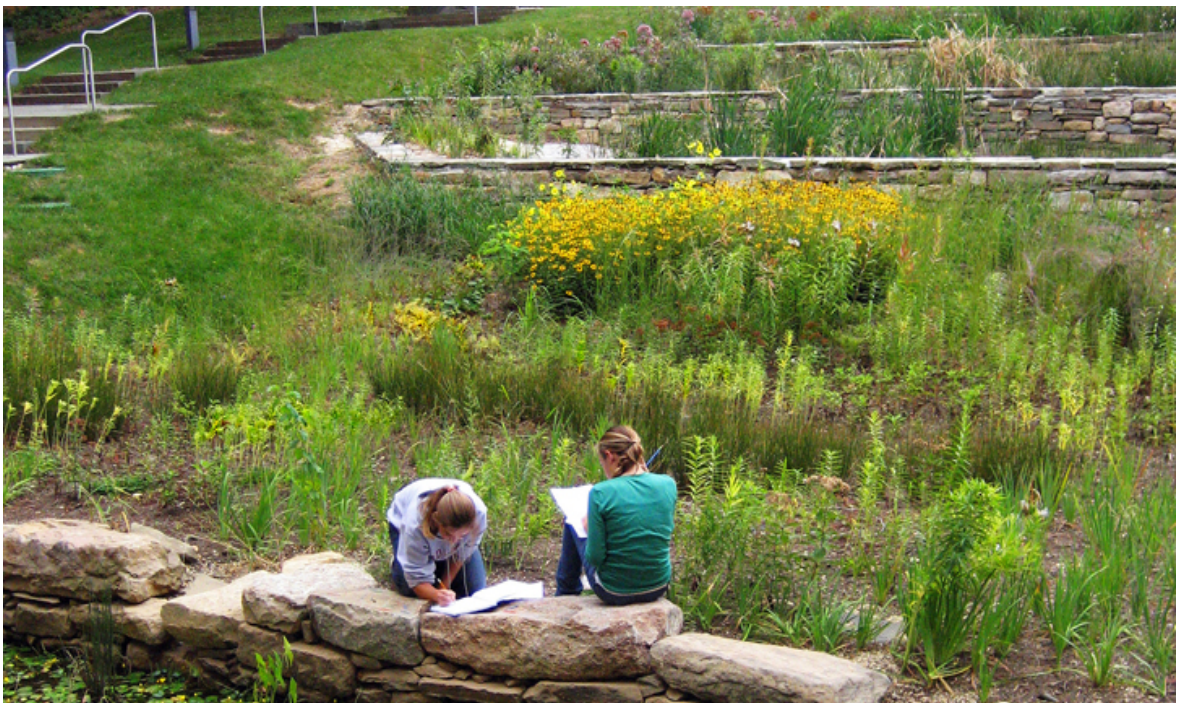
Figure 22. Recycled Stone Used for Terraced Wetland (Associates)
