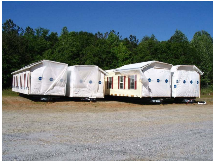
Figure 5.7. Tilt-up Roofs - Two double-section manufactured houses with tilt-up roofs. Once the house is installed on-site, the roofs will be jacked into place. The resulting higher roof pitch resembles that of a site-built house. (Photo by author)
