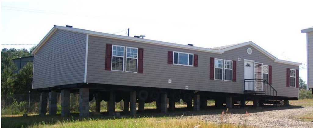
Figure 5.2. Typical manufactured home roof – 3:12 pitch (Photo by author)
