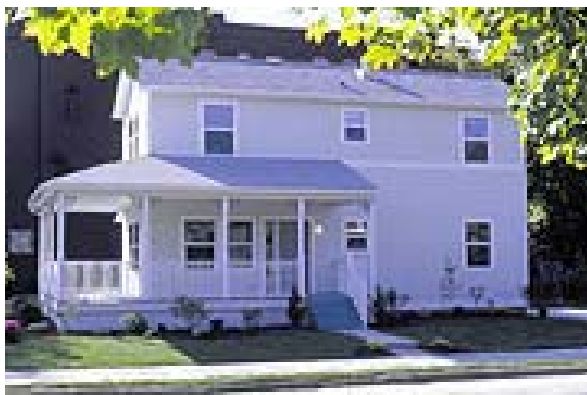
Figure 5.8. Demonstration Home 1 – A model manufactured home in Wilkinsburg, PA (MHI Website)
