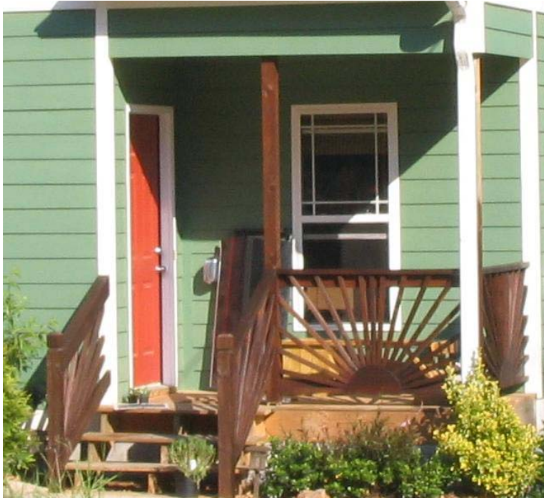
Figure 6.9. Incompatible ornament on this infill house includes “Craftsman” windows and radiating porch rails. (Photo by author)
