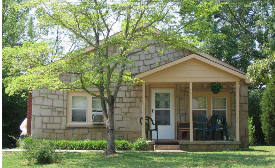
Figure 6.6. Typical front-gable house with front-gable portico (Photo by author)
