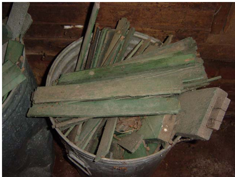
Figure 4.7 Broken and unattached louvers from Redcliffe Plantation. (Source: Author.)
