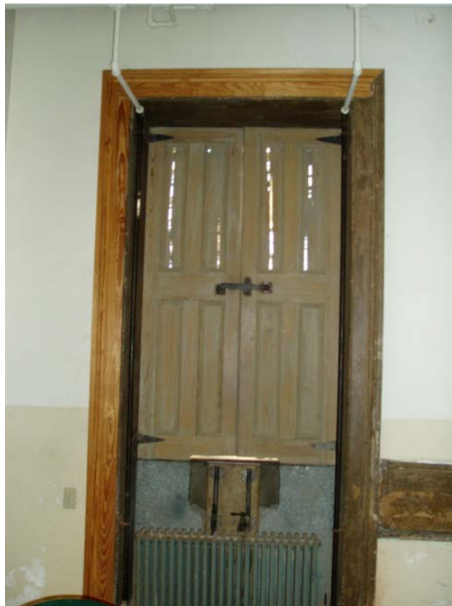
Figure 5.4 Paneled shutters located in the basement kitchen. (Source: Allison Moon.)
