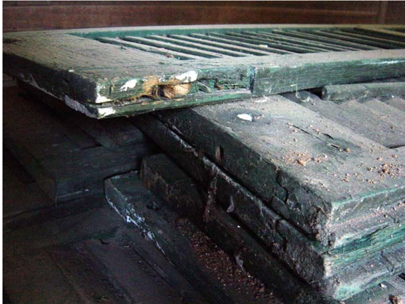
Figure 4.6 Shutters depicting mortise and tenon joints and previous repairs. (Source: Author.)
