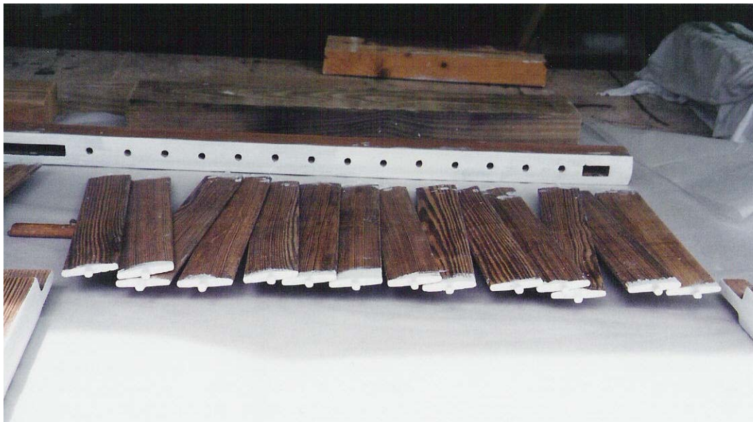
Figure 3.5 A dismantled shutter is ready to be reassembled. The frame employs a mortise and tenon joint while the louvers fit into holes drilled into the frame. (Source: Author.)
