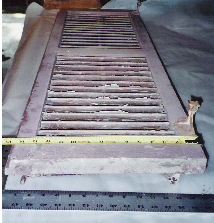
Figure 3.4 This shutter taken from Hollybourne Cottage still has its original hardware. (Source: Author.)
