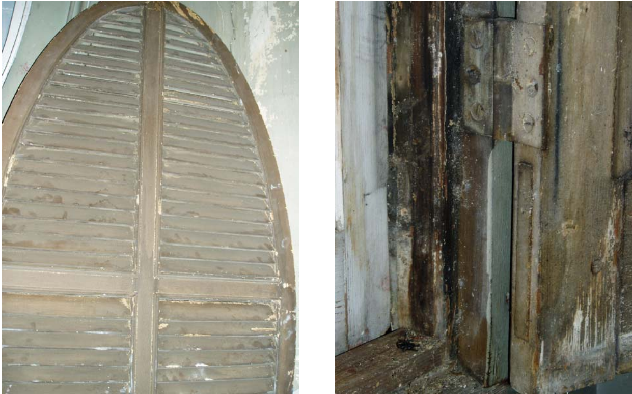
Figure 5.5 Water damage, rot, and paint failure are the most dominant conservation issues found on the cupola shutters. (Source: Allison Moon.)
