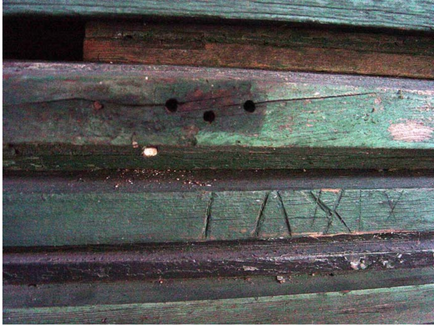
Figure 4.5 Roman numerals etched into the sides of the shutters are indicative of a numbering system. (Source: Author.)
