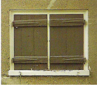
Figure 2.3 Board and batten shutters hung on iron strap hinges.(Source: Calloway, 114)
