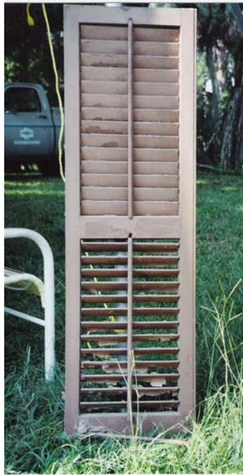
Figure 3.3 A sample shutter taken from the facade of Hollybourne Cottage. (Source: Author.)
