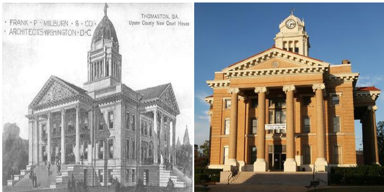
Figures 3.26 & 3.27 – The Historic Upson County Courthouse, Circa 1908 81 and Today 82
