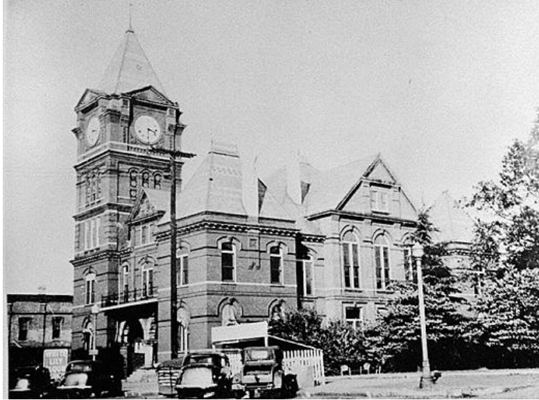
Figure 3.15 – Sumter County Courthouse, Circa 1944 64
