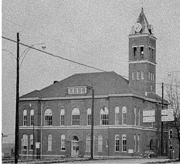
Figure 3.11 – Habersham County Courthouse, Circa 1953 60
