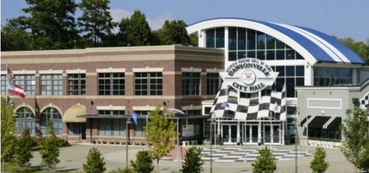
Figure 2.7 – City Hall, Dawsonville, Georgia
