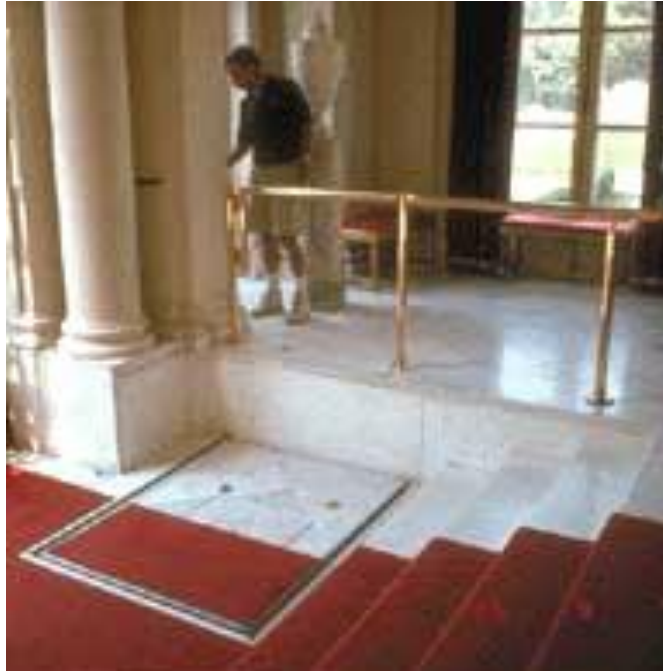
Figure 2.8 – ADA Compatible Entryway Using Historically Sensitive Materials 48
