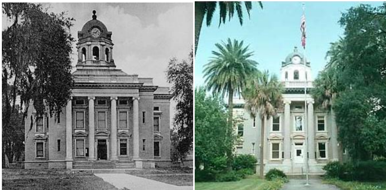
Figures 3.24 & 3.25 – The Historic Glynn County Courthouse (Date Unknown) 79 and Today 80
