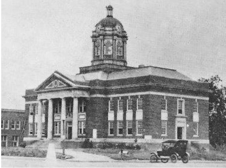
Figure 2.4 – The Neoclassical Style Barrow County Courthouse 35
