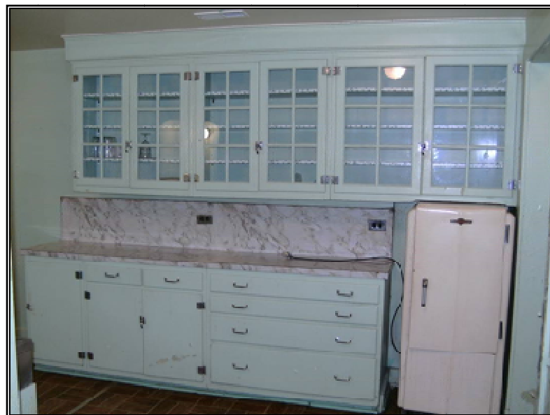
Figure 6.25: Butler's pantry north cabinet as built by Curtis Woodwork. Note: Base cabinet was built as designed but, during installation, the left cabinet was dropped and the entire unit moved to the left to accommodate the pantry refrigerator. The wide drawers to the right are for flat linen storage
