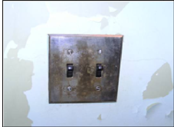
Figure 6.29: Typical chrome plated switch plate cover in the service wing
