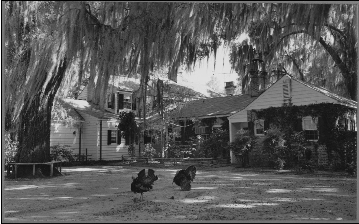
Figure 6.31: Exterior view of the north wall of the service wing dated 1952. Window air-conditioning unit can be seen in the upper portion of the kitchen window.
