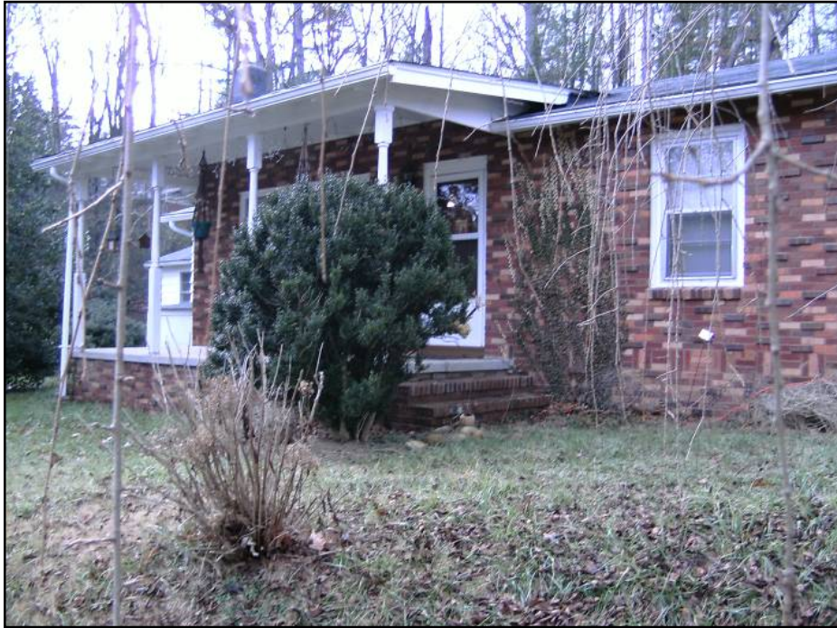
Figure 6.18: Glenwood Road - facade
