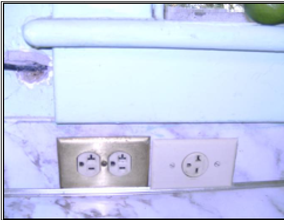
Figure 6.30: Kitchen north wall outlets. Neither of these is original. The one on the left is a 1950s era grounded outlet. The one to the right is a 1940s era 220 v. outlet that serviced the first window air-conditioner in the house.
