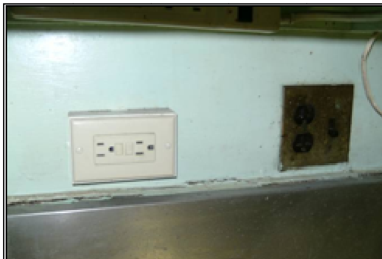
Figure 6.27: South wall of kitchen – original two-gang outlet with switch for the light over the sink with a chrome-plated cover to the right. The outlet to the left is ca. 1980 and was placed to service a microwave oven.
