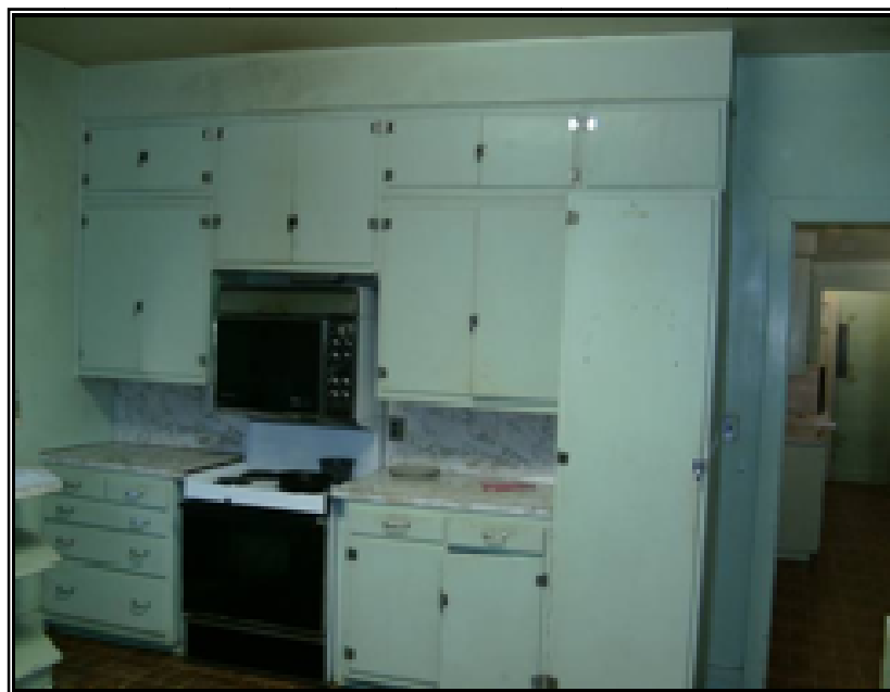
Figure 6.34: Kitchen east wall cabinets as built by Curtis Woodwork. The cut for the stove was made at some point during the 1960s. The Formica on the counters and back splash cover the original white oak material.
