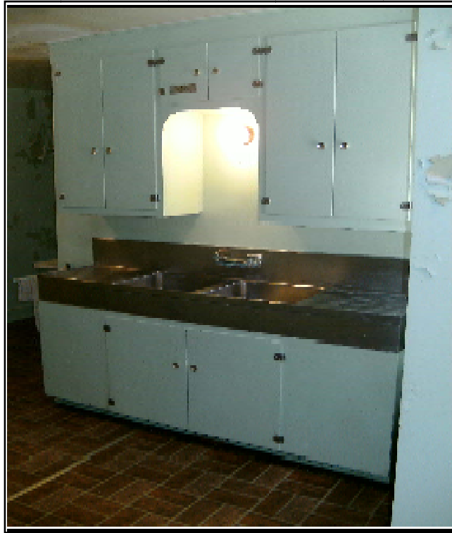
Figure 6.26: Monel metal sink in butler's pantry. This sink originally appeared as wall-mounted with no cabinetwork. The current cabinetwork is of low quality and was added at a later unknown date.
