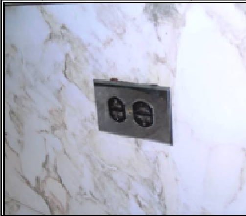
Figure 6.28: Typical chrome-plated outlet cover in the service wing
