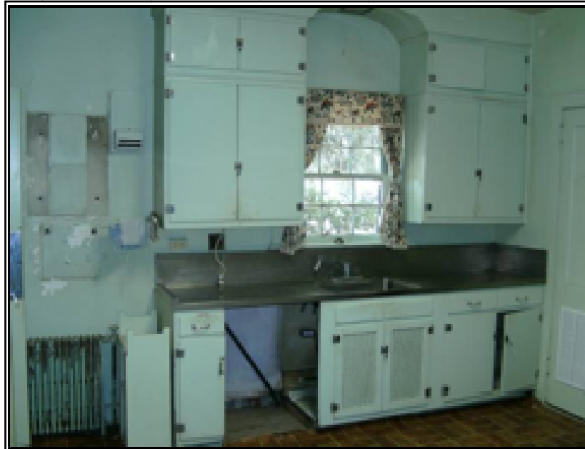
Figure 6.33: Kitchen south wall cabinets as built by Curtis Woodwork. Features include Monel metal countertop, vent grill in doors below sink, and extremely fine chrome plate on brass cabinet hardware. The cut in the base cabinet to the left of the sink is from a 1960s era dishwasher installation.
