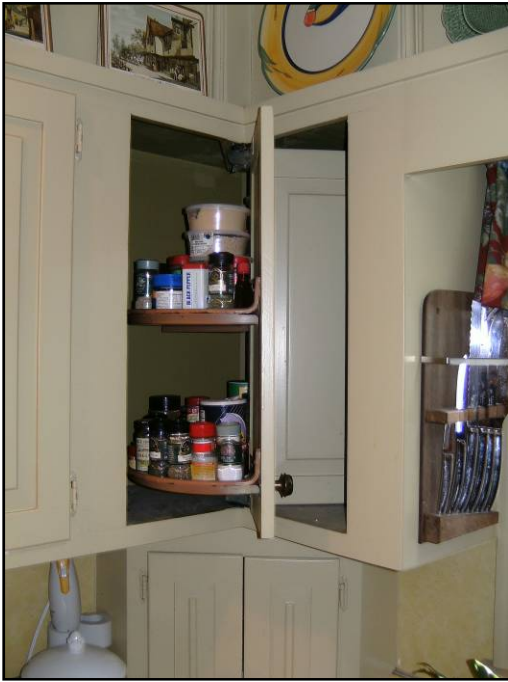
Figure 6.13: Close-up of “lazy-susan” cabinet in corner – an innovative feature in high-end cabinetry of the period
