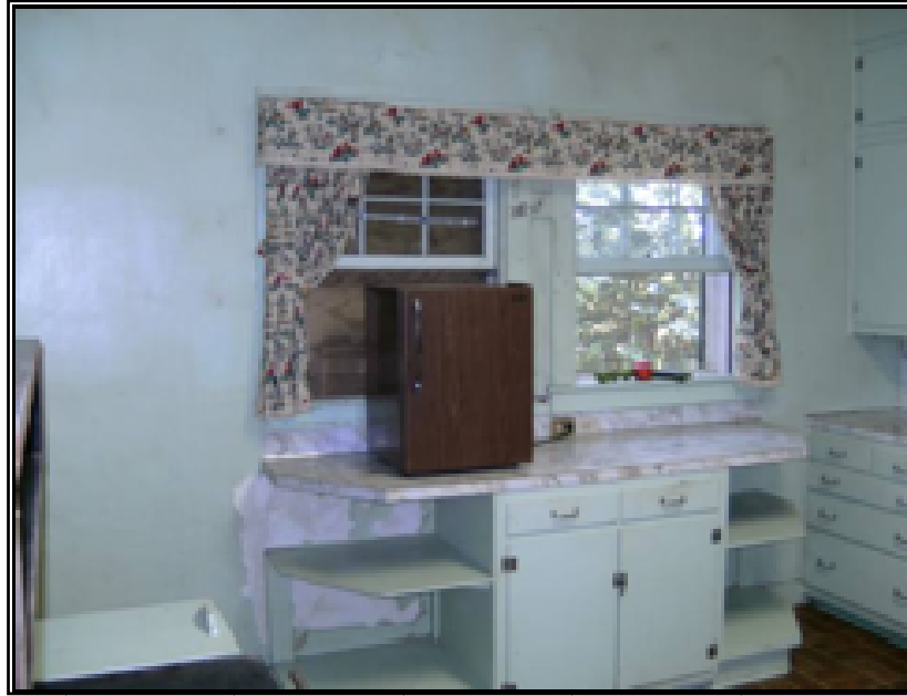
Figure 6.35: North wall cabinet added sometime during the 1960s. The center portion is made from the section removed from the east wall base cabinet.
