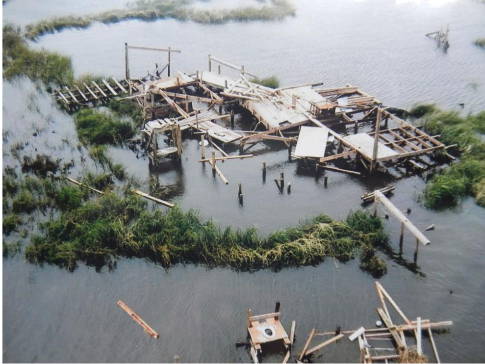
Figure 95: Threats to preservation come from storms, flooding, and coastal erosion. Here The Delacroix Hilton is seen after being washed away by a storm (photo courtesy of Kerryn Liebke)
