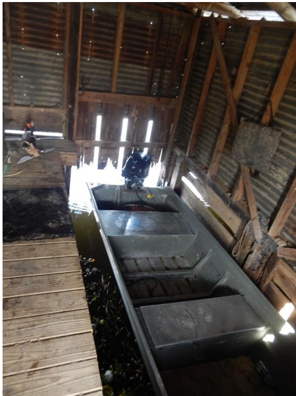
Figure 39: The interior of the boathouse at The Red Camp (photo by author)
