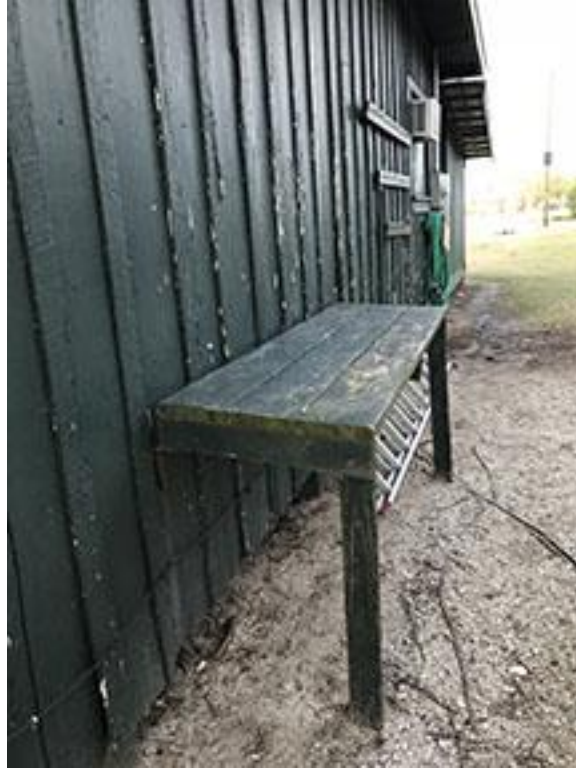
Figure 23: The original cleaning table is still attached to the wall on the east side of the primary camp building
