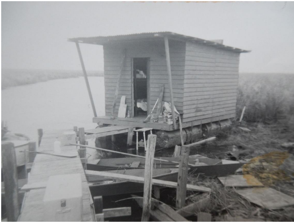
Figure 80: The camp under construction in 1955 (photo courtesy of Kerry Liebkeman)
