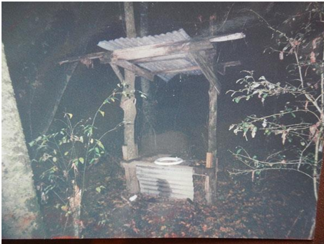
Figure 64: Until 1995, there was no interior bathroom at Hard Times Camp so this outdoor toilet made do (photo courtesy of Rachal family)
