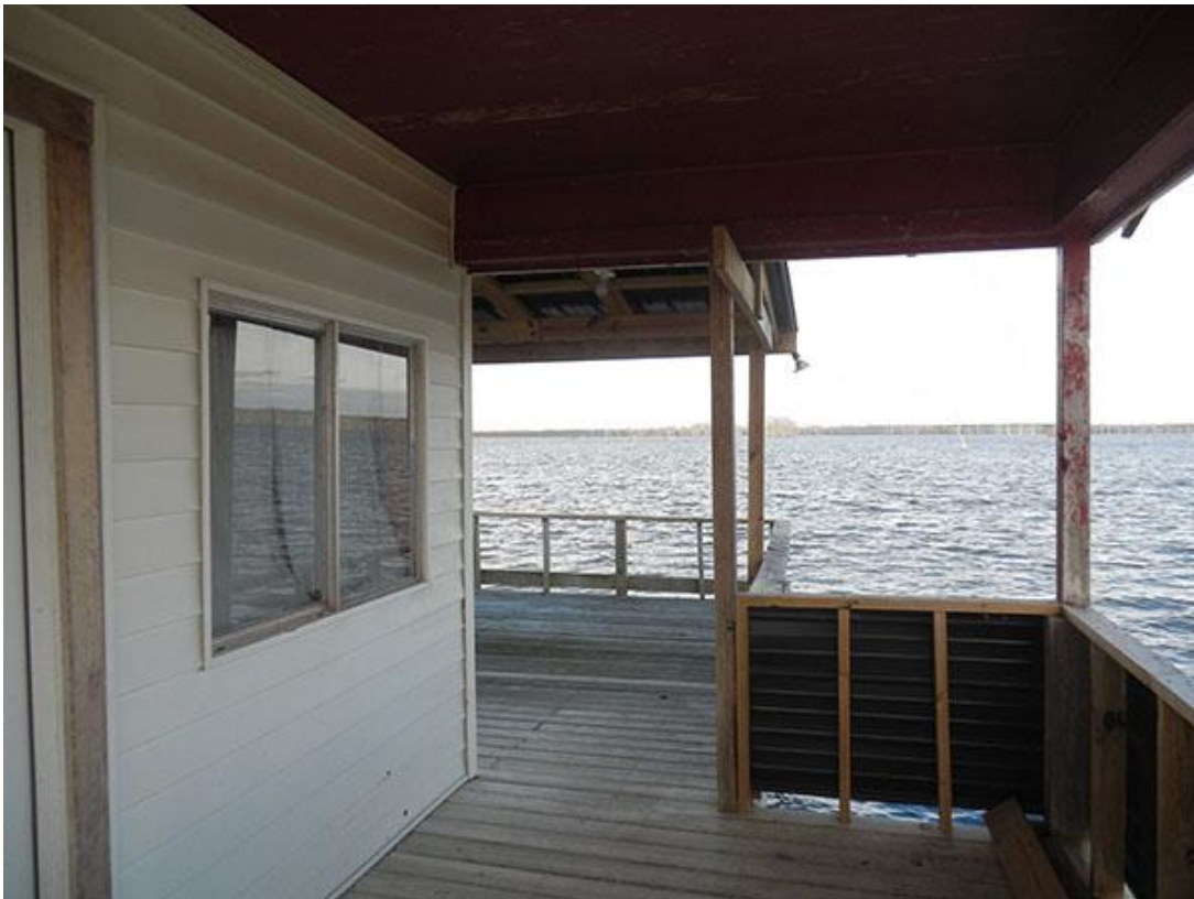
Figure 40: The porch wraps around the east and north elevation (photo by author)
