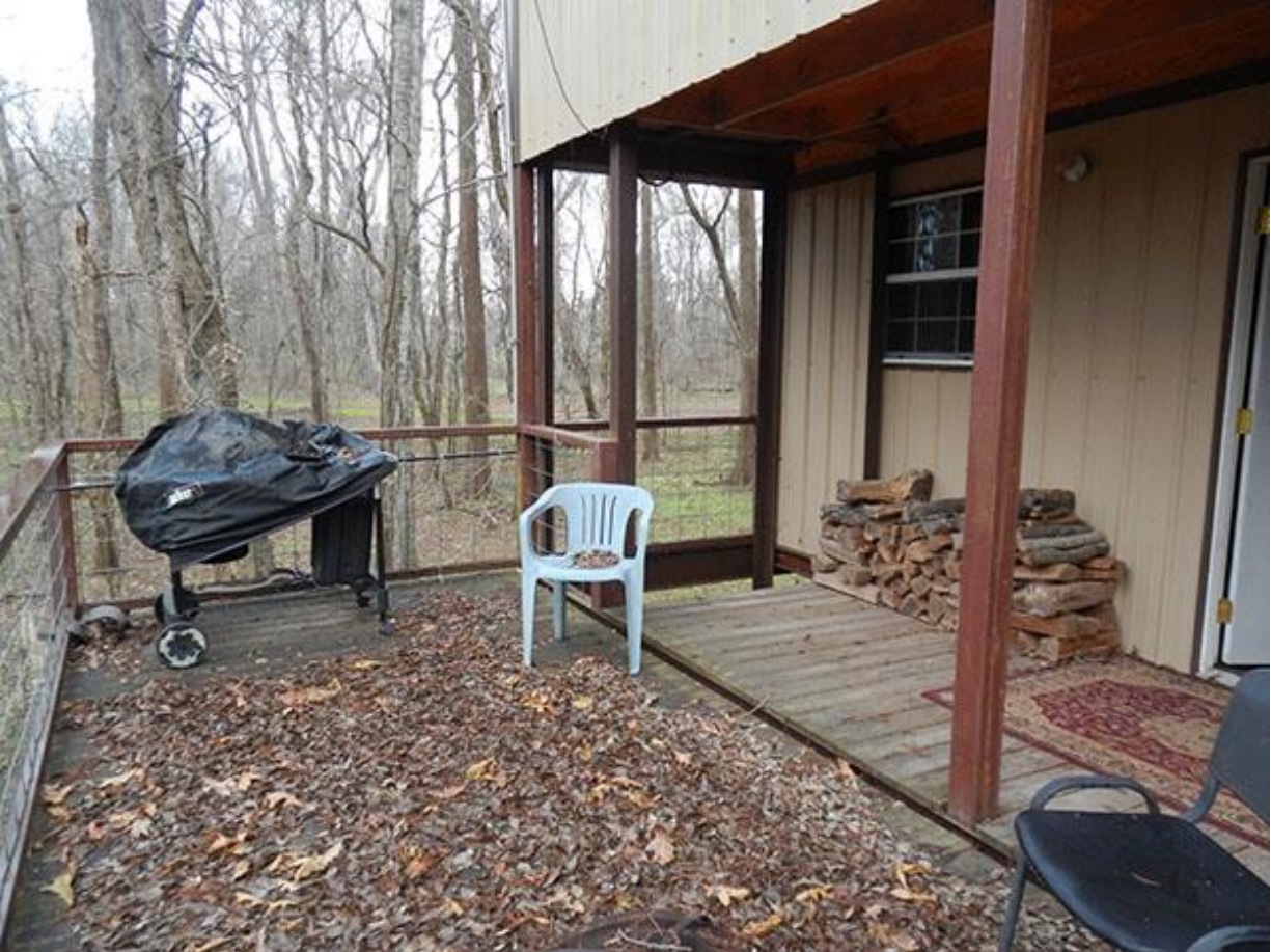
Figure 59: The porch on the north elevation is the primary outdoor space (photo by author)
