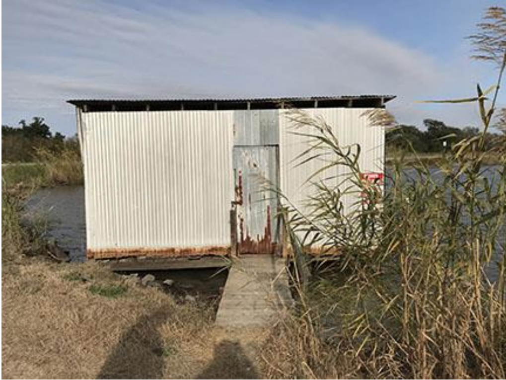
Figure 21: The southwest elevation of the boathouse (photo by author)
