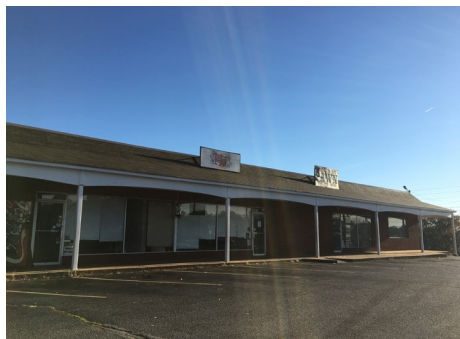
108 Gaines School Rd.
