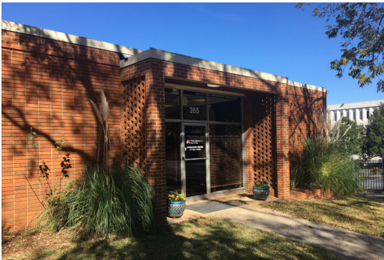
Figure 6.25: 265 E Hancock Ave.
