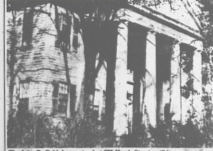
The John B. Cobb house stood at 575 Harris Street until it was torn down and replaced by the building now housing Magic Years of Learning Day Care Center.
