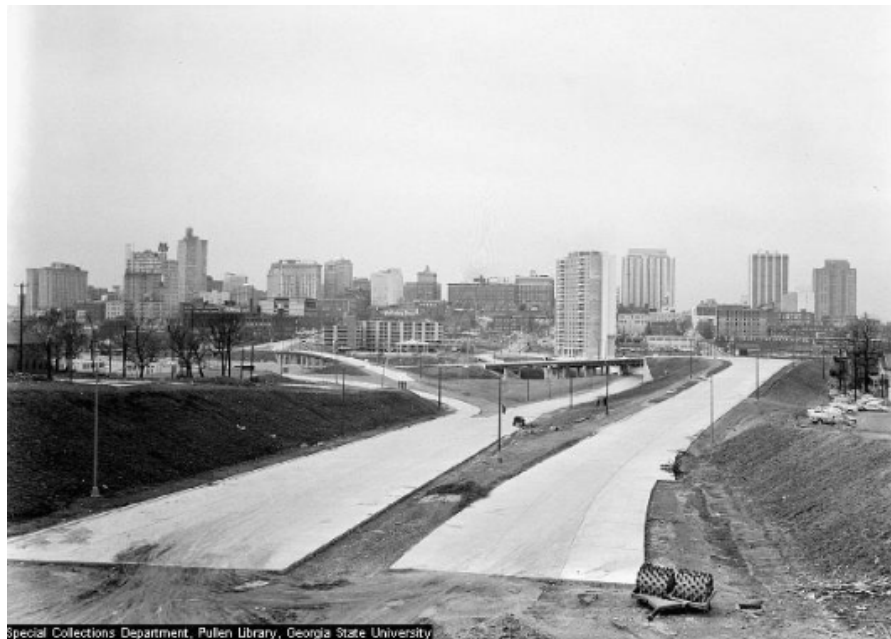
Figure 3.17: Highway construction underway in Atlanta.
