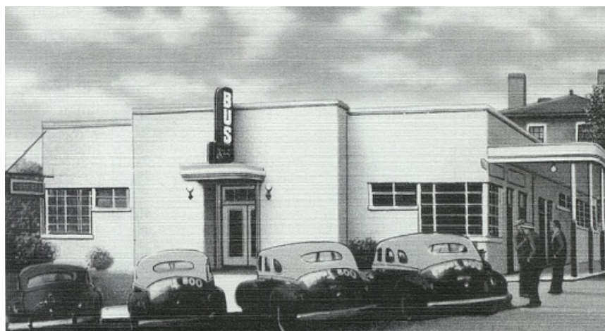
Figure 3.13: The Union Bus Terminal at 220 W. Broad St. was completed by 1940. True to the architecture of the era, Greyhound Bus corporate design, and the spirit of transportation, the terminal shows Streamline Moderne style.
