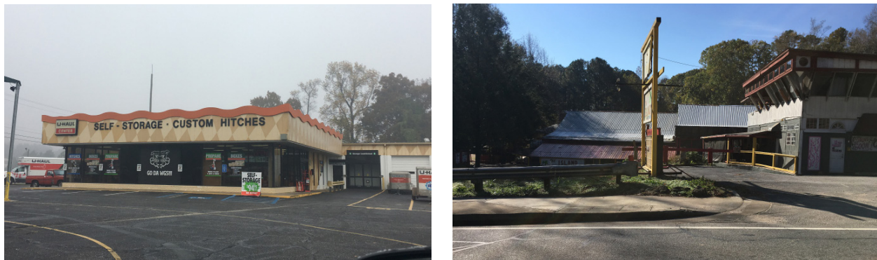
Figure 6.18: Both buildings have loss of integrity. 2900 Atlanta Highway (left) shows planned loss whereas 215 Tallassee Rd. (right) shows more unplanned, ad hoc loss.
