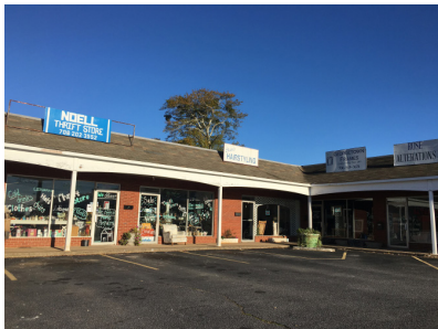
108 Gaines School Rd.
