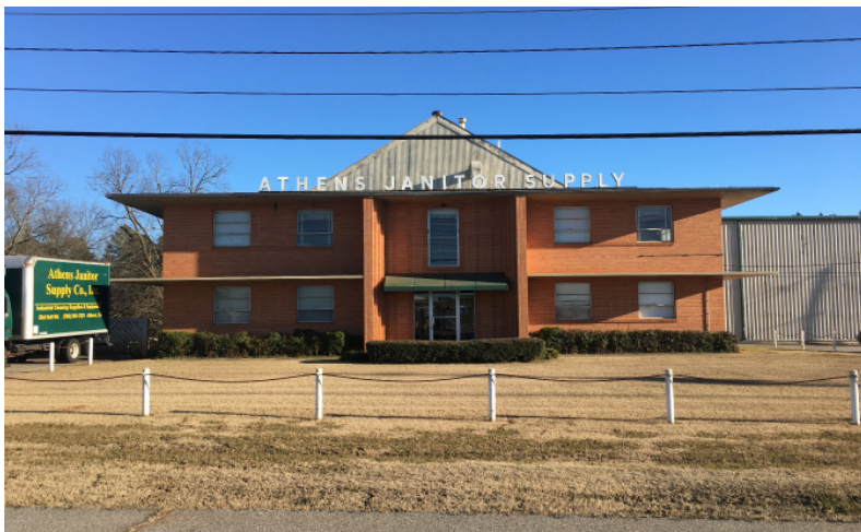
Figure 6.27: 900 Old Hull Rd.
