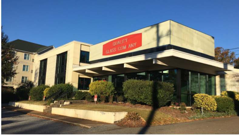
Figure 6.26: 234 Old Epps Bridge Rd.
