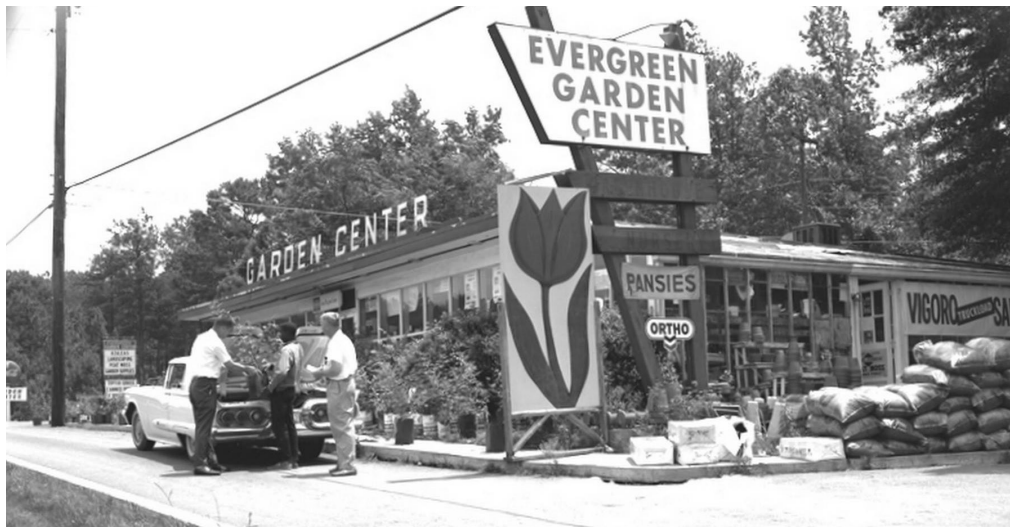
Figure 3.28: Examples of businesses being designed in the commercial architecture of the mid-century with canted glass, brick veneer, visual fronts, and angular signs. Arctic Girl on Broad St. (top left); Phillips 66 on Oconee St. (top right); Grant's department store in Beechwood Shopping Center (middle); Evergreen Garden Center on Atlanta Highway (bottom)
