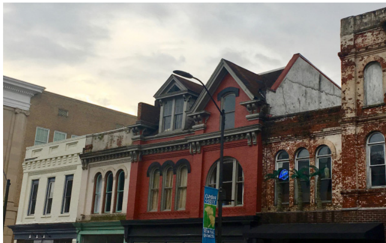
Figure 6.5: Rooflines of traditional connected storefronts, such as these in downtown Athens, were often more ornamental than functional, whereas modern storefronts utilized rooflines for both ornamental and functional purposes.
