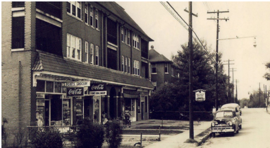
Figure 3.10: The commercial buildings at Five Points were of more sturdy construction compared to the "taxpayers" at Normaltown, with apartments above the storefronts.
