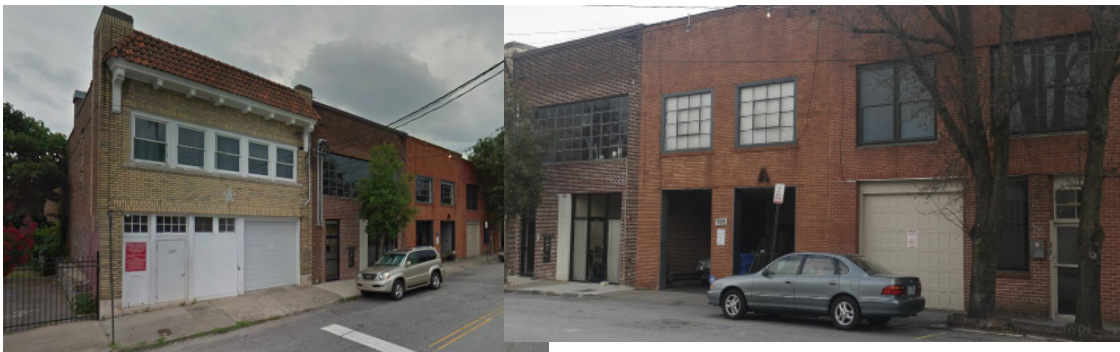
Figure A-38. 132- 136 Walker Street.
