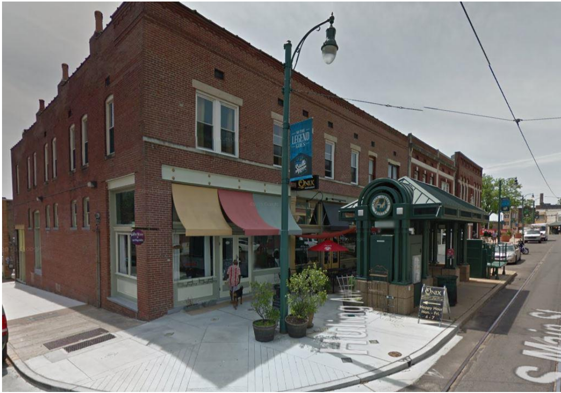
Figure 12. 410 South Main Street (Google street view).
