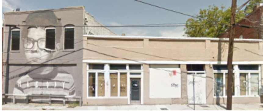
Figure A-22. 33 Walker Street (Google street view).
