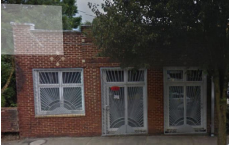
Figure A-34. 211 Walker Street (Google street view).
