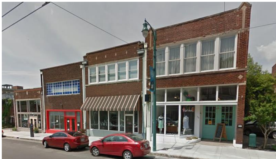
Figure 14. 509-515 South Main Street (Google street view).
