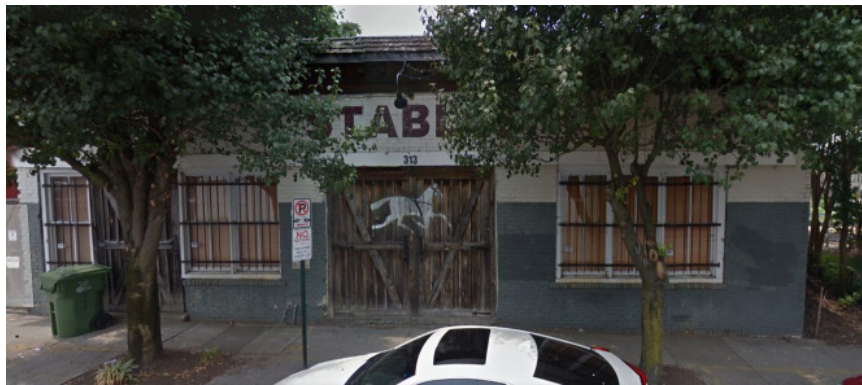
Figure A-24. 313 Walker Street (Google street view).
