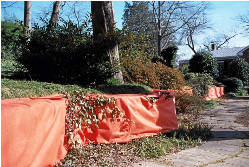
Figure 44: Orange Wall. View from North Side. February 11, 2007.
