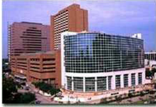
Figure 2.2 Modern Hospital, Texas Heart Institute, Houston Texas
