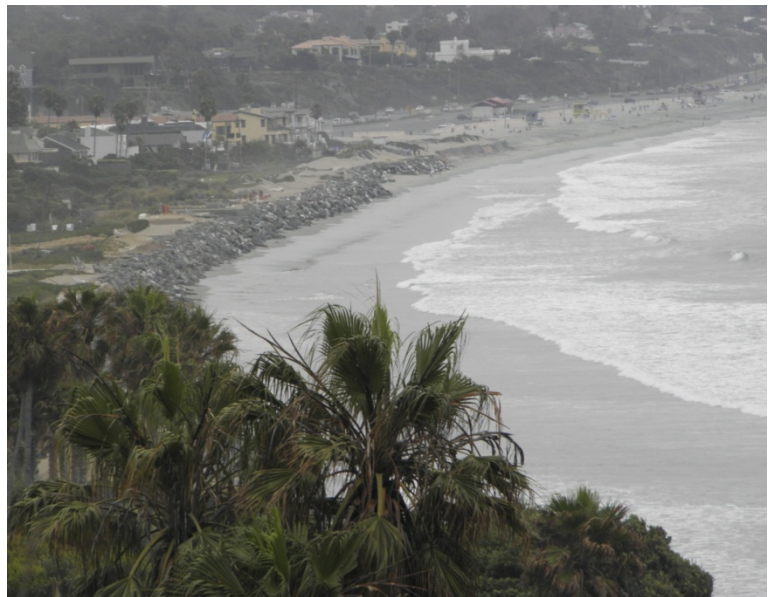
Figure 7.12 Rock revetments in Broad Beach, 2011. Photo: M.Palma
