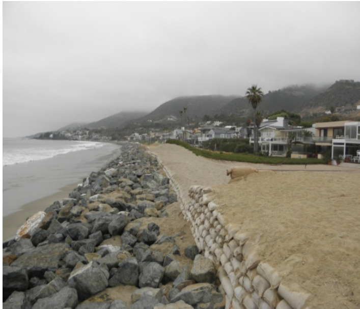
Figure 7.11 Rock revetments in Broad Beach, 2011. Photo: M.Palma
