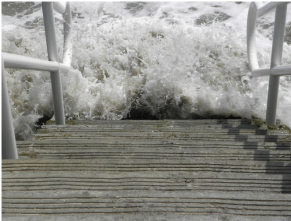
Figure 7.15a Water covering bottom steps of access way. Photo: M.Palma
