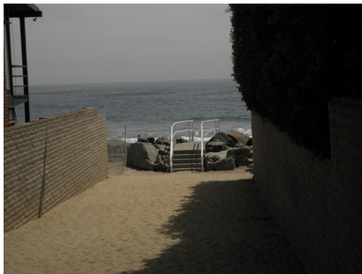
Figure 7.14 Concrete steps. Photo: M.Palma
