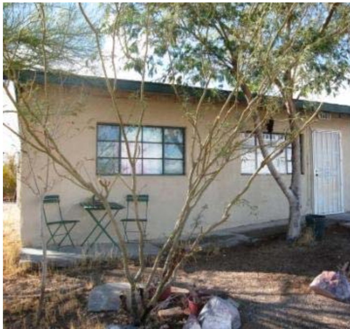
Figure 2.11 My home, one of the early adobe houses built to stay warm in the winter and cool in the summer. The mesquite tree in the foreground provided welcomed shade during the hot summer months.
