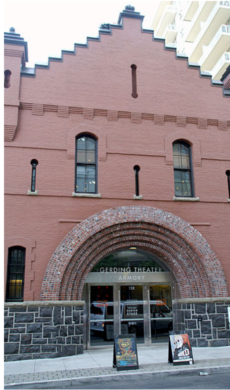
Figure 6.4 Gerding Theater (Front Doors). 143
