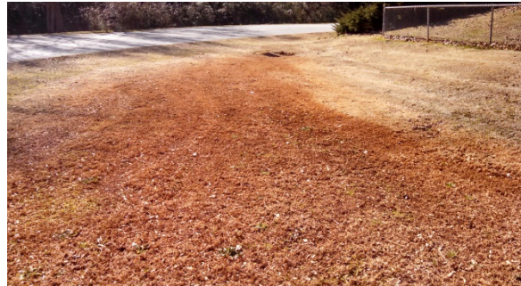
Figure 10: Photo of the lower portion of the intramural fields swale. Sediment is visibly streaked across the grass.
