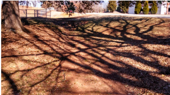
Figure 9: Photo of the upper portion of the intramural fields swale. The swale is shaded and grass coverage is sparse.
