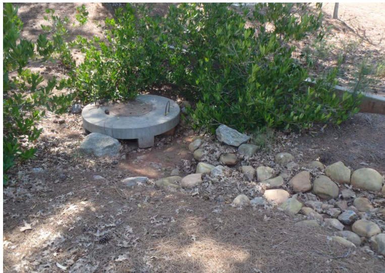
Figure 14: Photo of a storm inlet near the tennis courts. This outlet structure in one of the existing rain gardens is not elevated, and thus allows for no ponding before the SCM overflows. Better function could be achieved if the structure's inlet elevation were raised.
