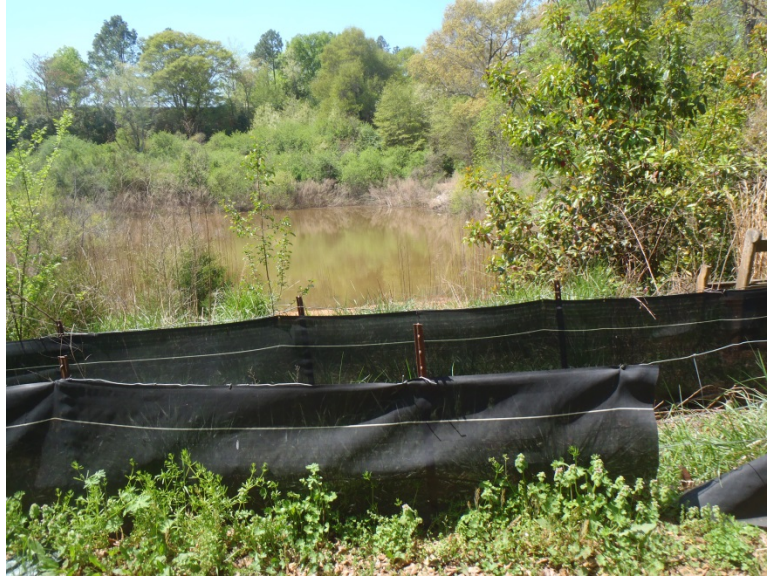
Figure 17: Photo of silt fencing around Parvo Pond.
