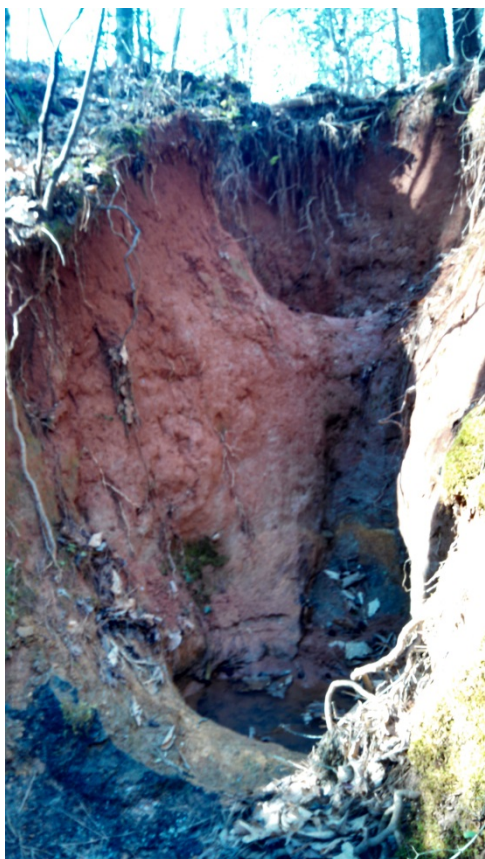
Figure 12: Photo of the eroded gully where runoff from Family Housing discharges.
