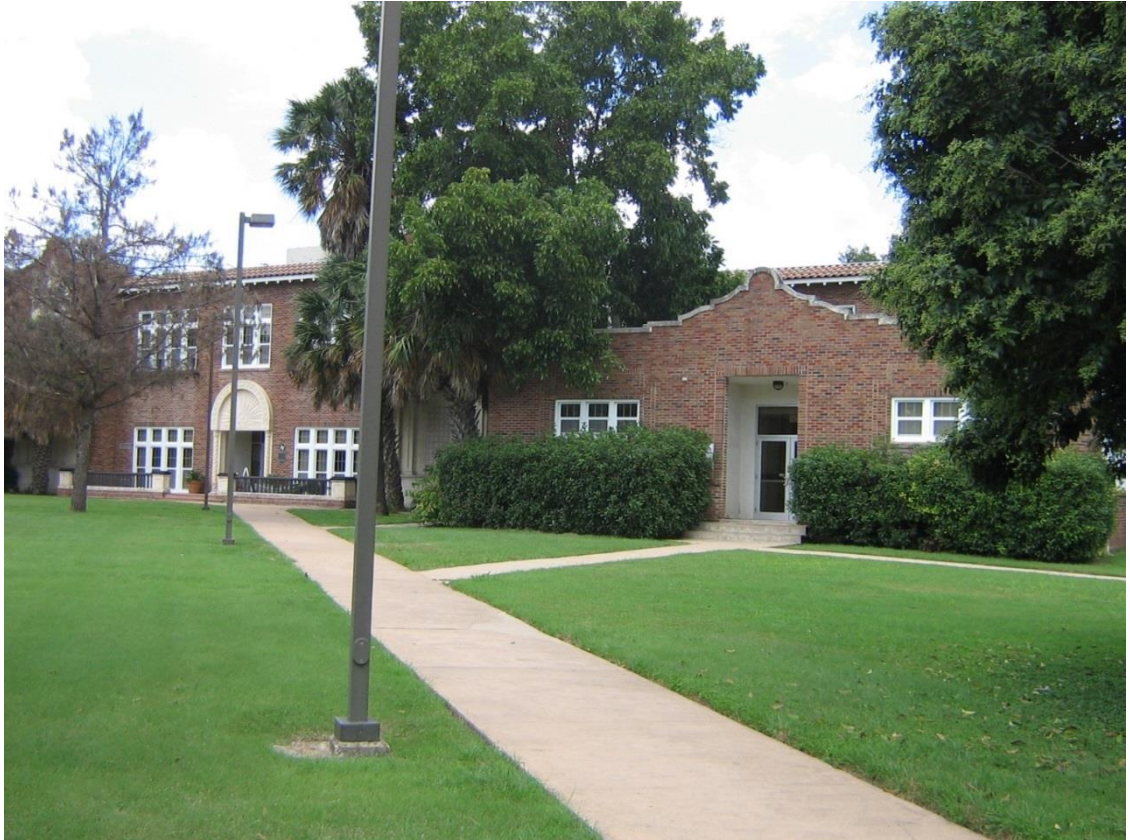
Figure 8.5: The approach to the historic school has the obvious addition of modern lighting and new pavement, but otherwise is preserved. The district plans to remove some of the trees and landscaping close to the building that obscures the historic architecture. (Photo courtesy of Georgetown ISD)
