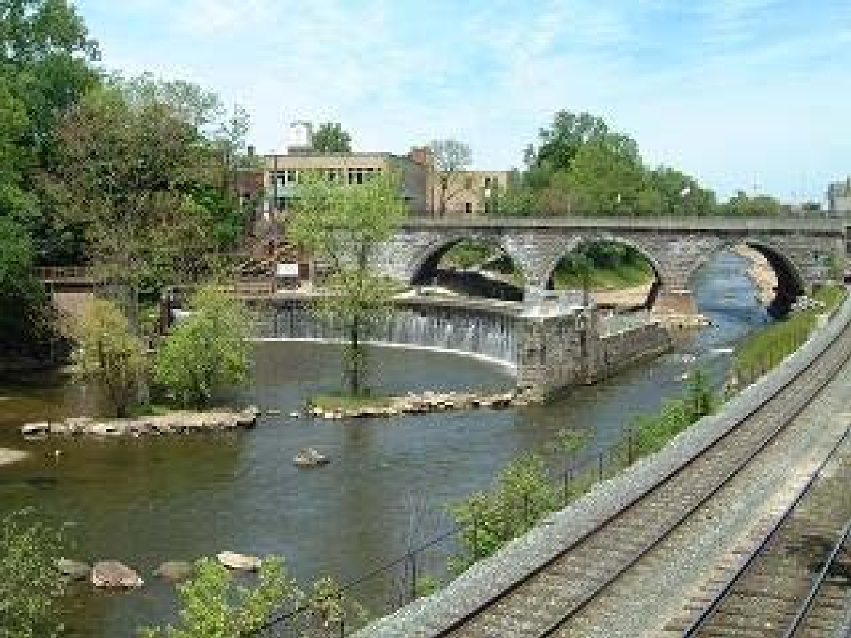
Figure 26. Kent Dam after partial removal.
