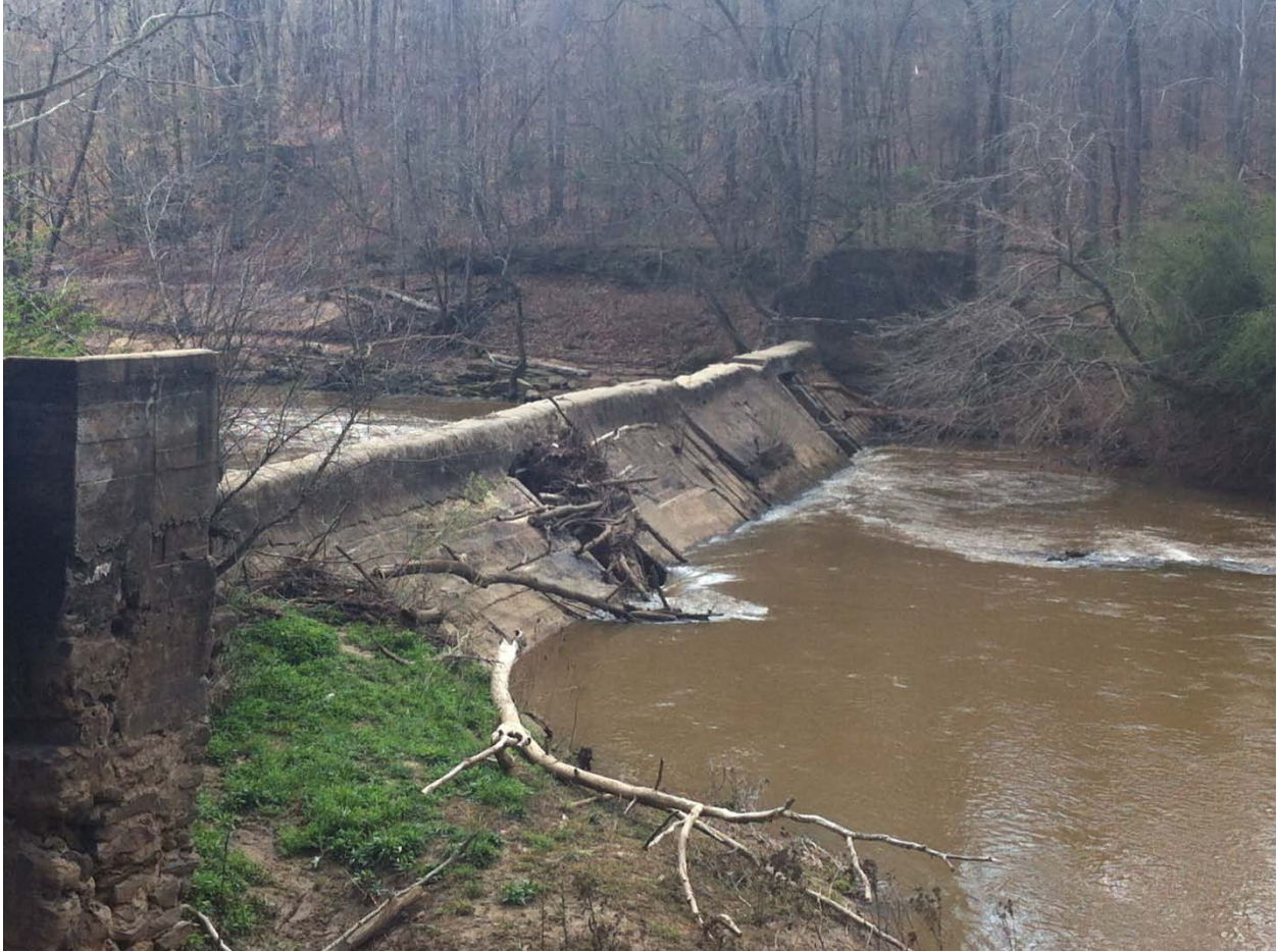
Figure 12. Upstream face of Whitehall Dam.
