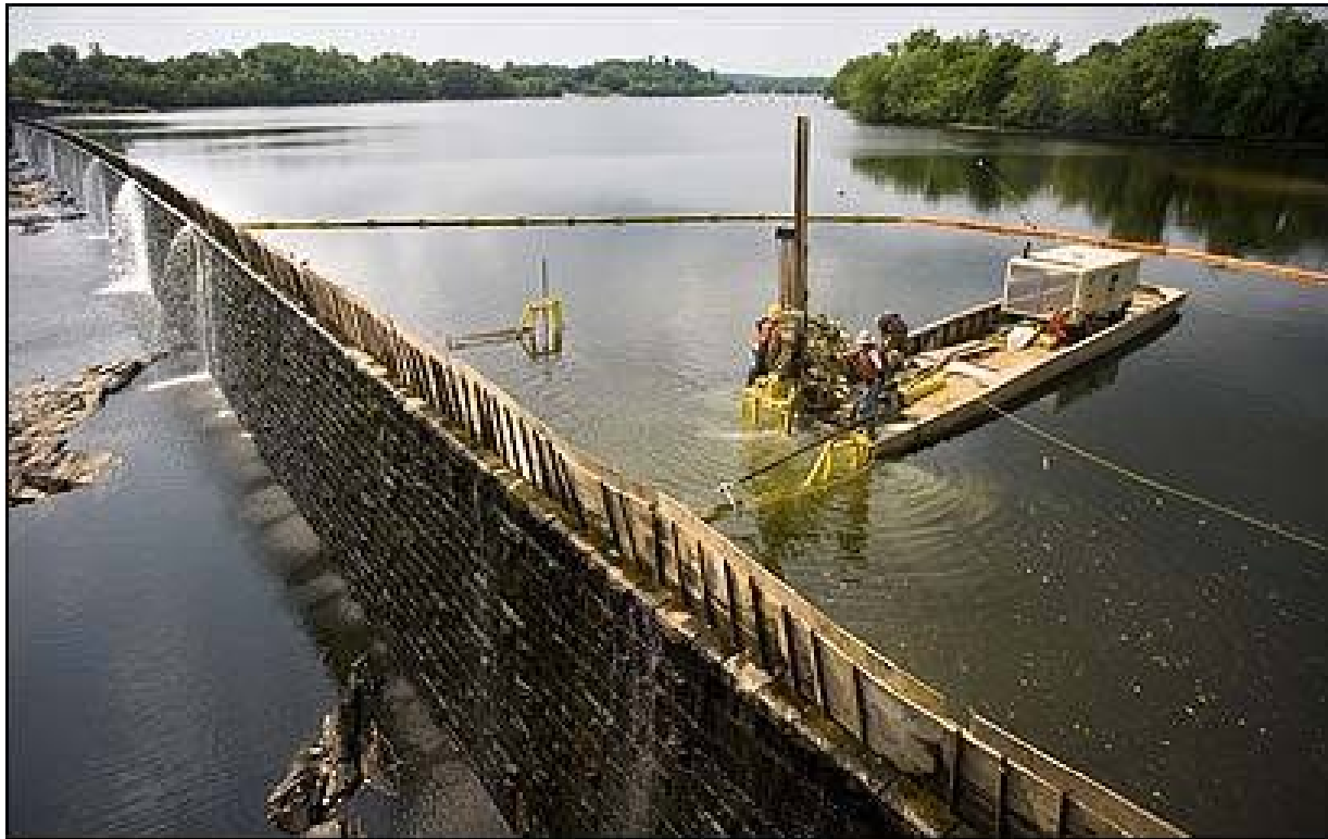
Figure 16. Flashboards atop a masonry dam.
