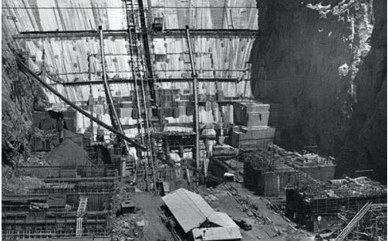
Figure 8. Hoover Dam construction.
