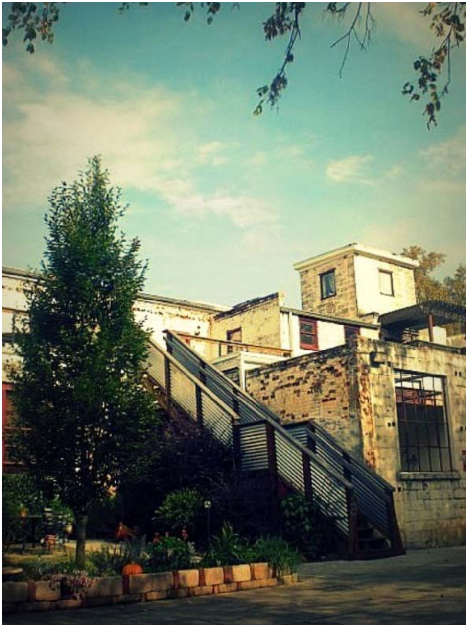
Figure 13. Current usage of Whitehall Mill.
