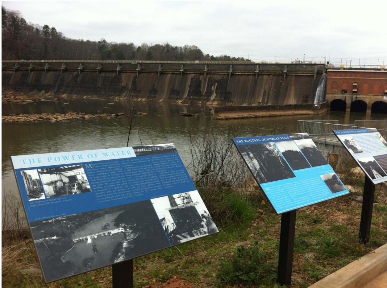
Figure 22. Interpretive signage at the base of Morgan Falls Dam.
