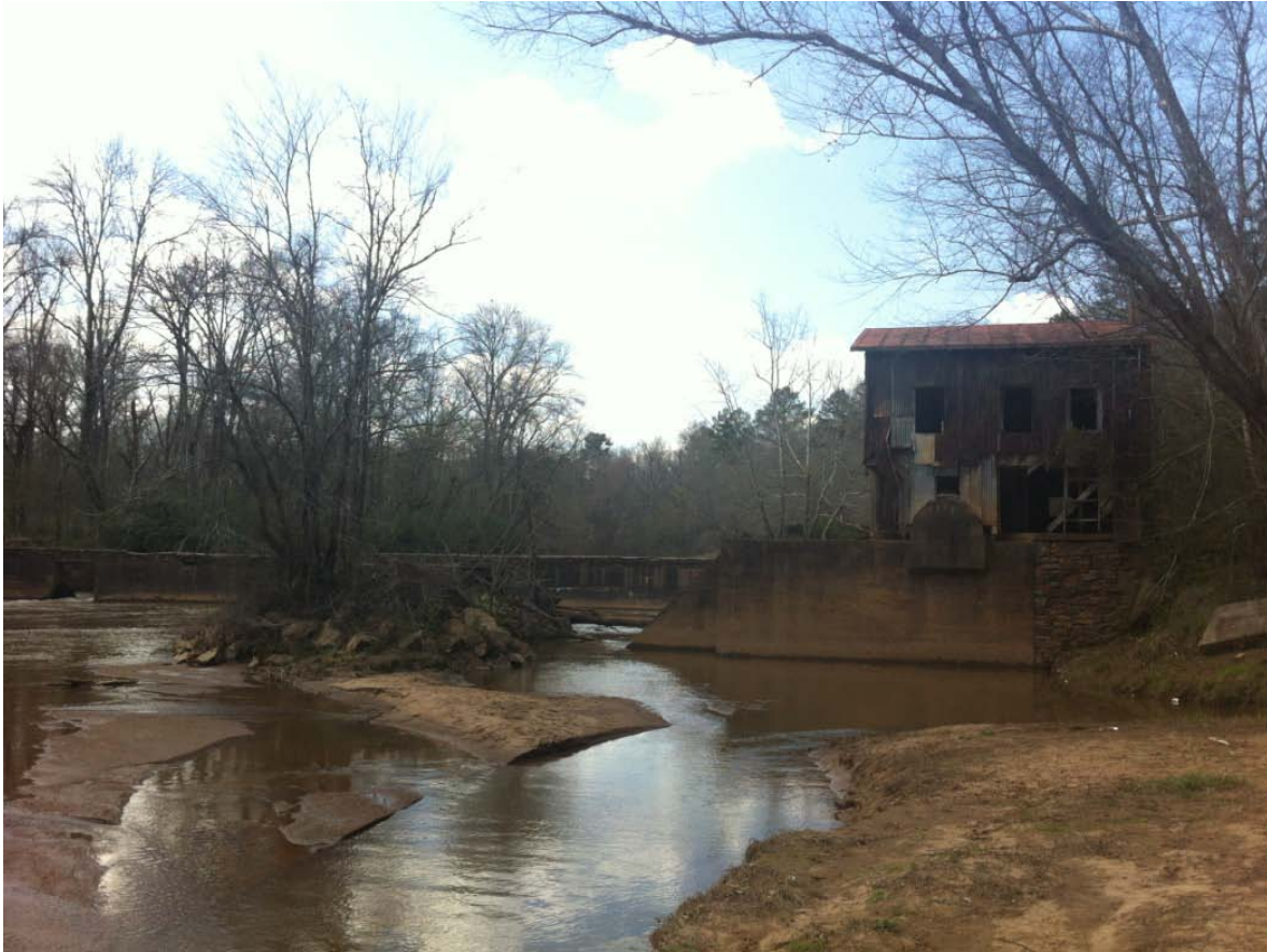
Figure 14. Current condition of Whitehall Dam.
