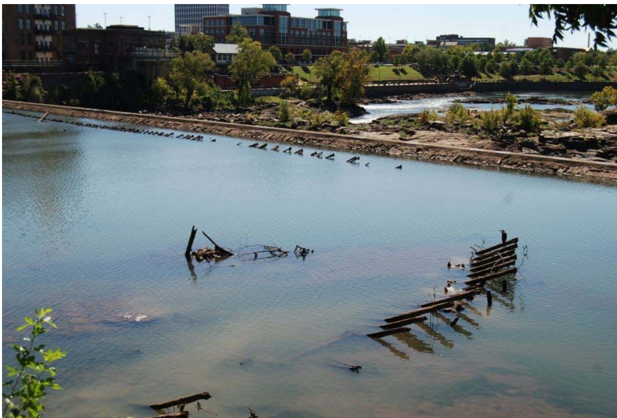
Figure 19. Remnants of wooden crib dams upstream from Eagle-Phenix dam.
