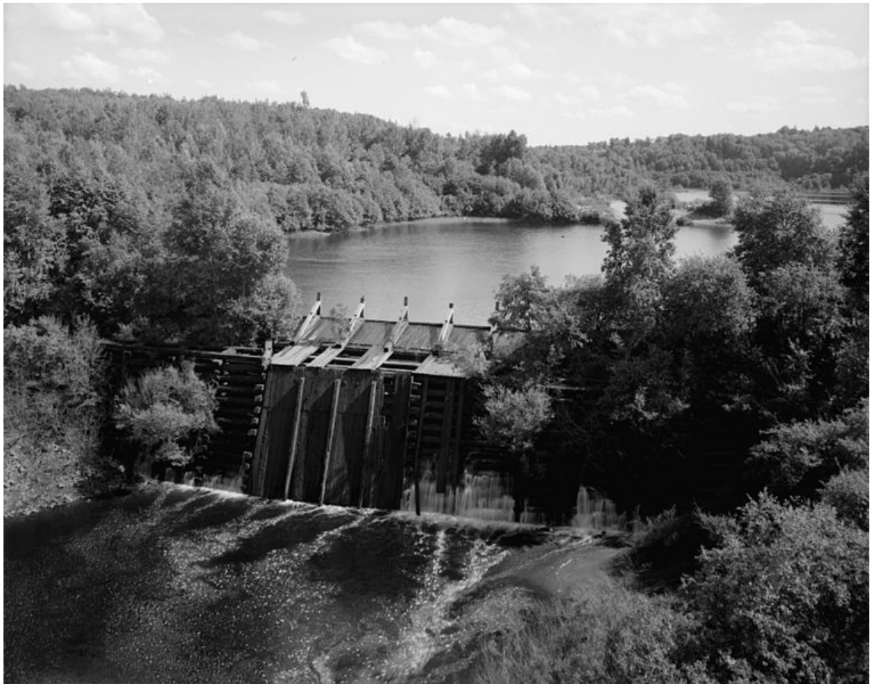
Figure 3. Timber crib dam.
