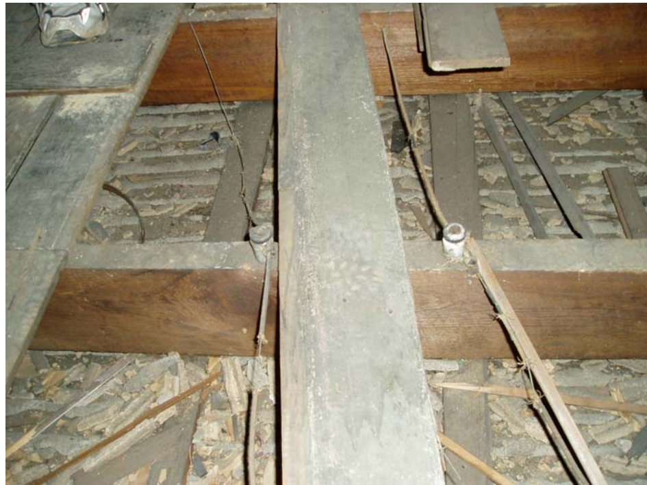
Figure 13 Remnant of 1903 knob and tube wiring. Photo by author.
