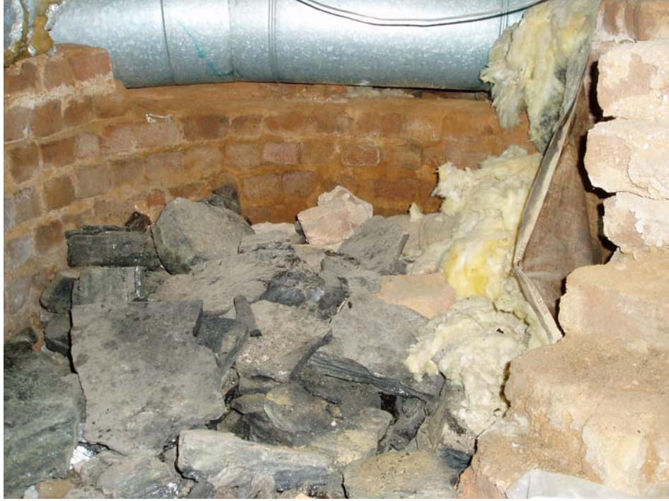
Figure 25 Old brick well under house. Photo by author.
