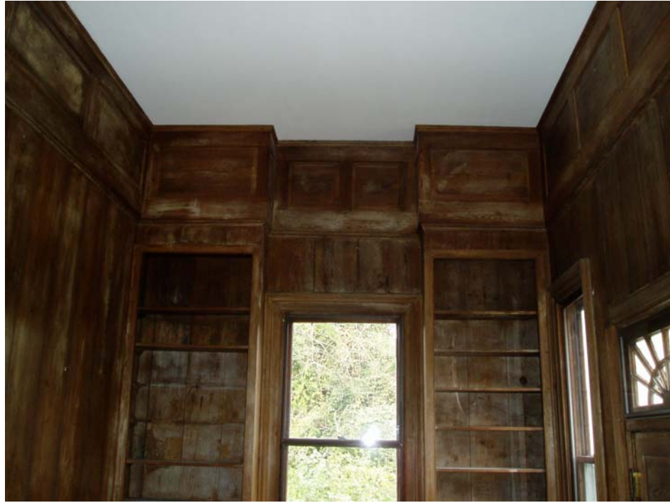
Figure 12 Detail of woodwork in library. Photo by author.
