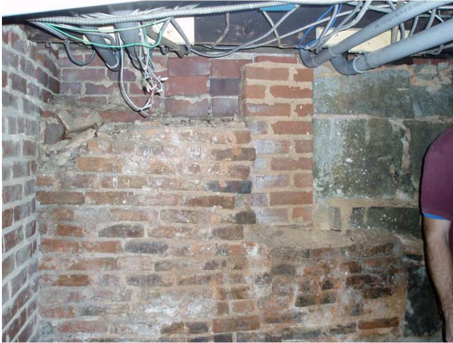
Figure 6 Irregular foundation under kitchen. Photo by author.
