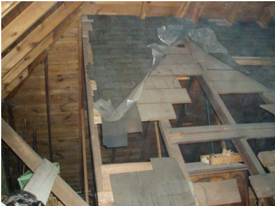
Figure 5 Remnant of dormer in 1903 roof. Photo by author.
