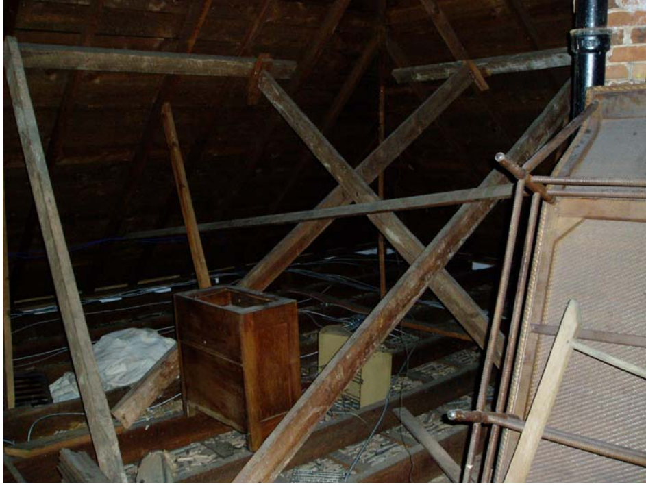
Figure 15 Ad hoc roof reinforcement with old timber. Photo by author.
