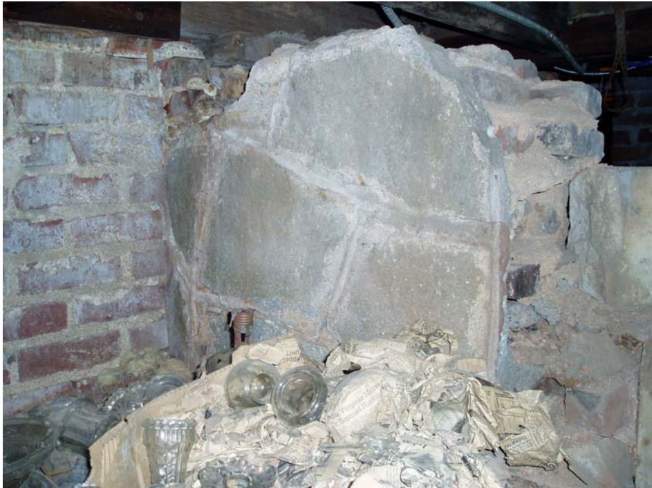
Figure 16 Beaded mortar joint on foundation remnant. Photo by author.
