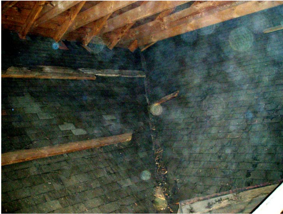
Figure 4 Remnant of 1903 intersecting roof line. Photo by author.
