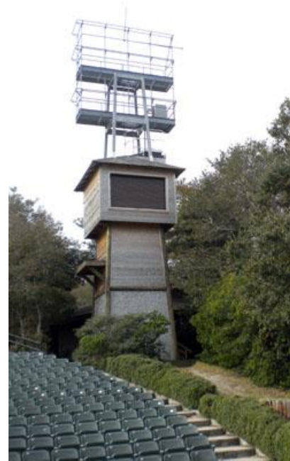
Figures 5.6: New Lighting Tower
