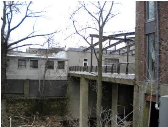
Figure 5.46: Bridge that the Ubu Roi technical crew strung extension cords across to bring electricity to the site.
