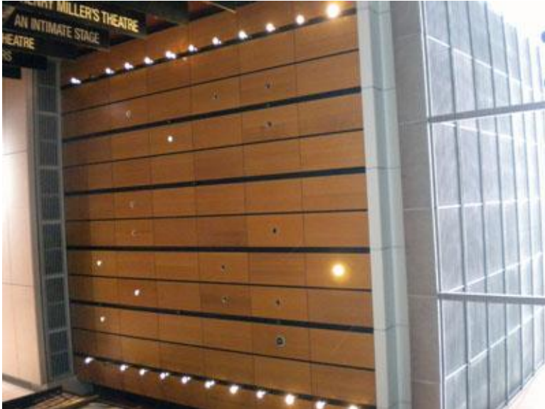
Figure 5.36: Ceiling made of bamboo paneling
