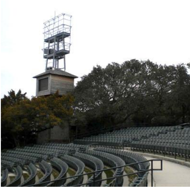
Figures 5.5: New Lighting Tower
