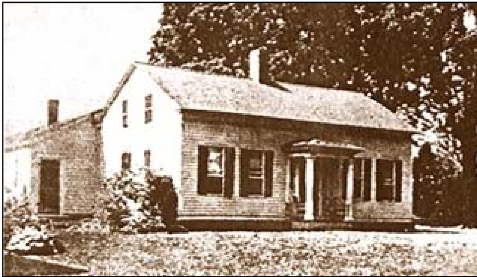
Figure 5: Historic photograph of Ames house, date unknown (Photo courtesy of Oswego State University of New York; http://www.oswego.edu/ugrr/ames.html )
