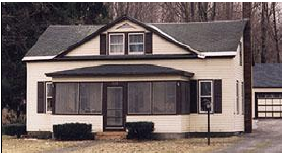
Figure 6: Photograph of Ames house with alterations, 1999 (Photo courtesy of Oswego State University of New York; http://www.oswego.edu/ugrr/ames.html )
