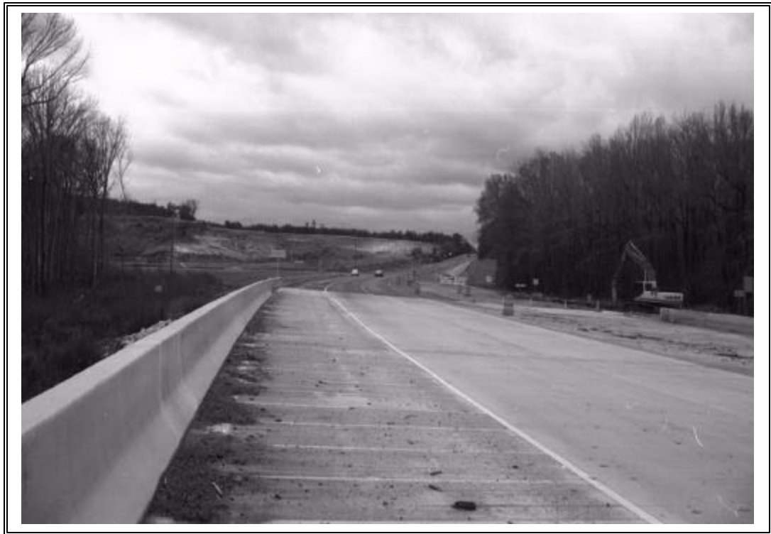
Figure 7.3: Along the route, view of highway improvements at McBeans Creek
