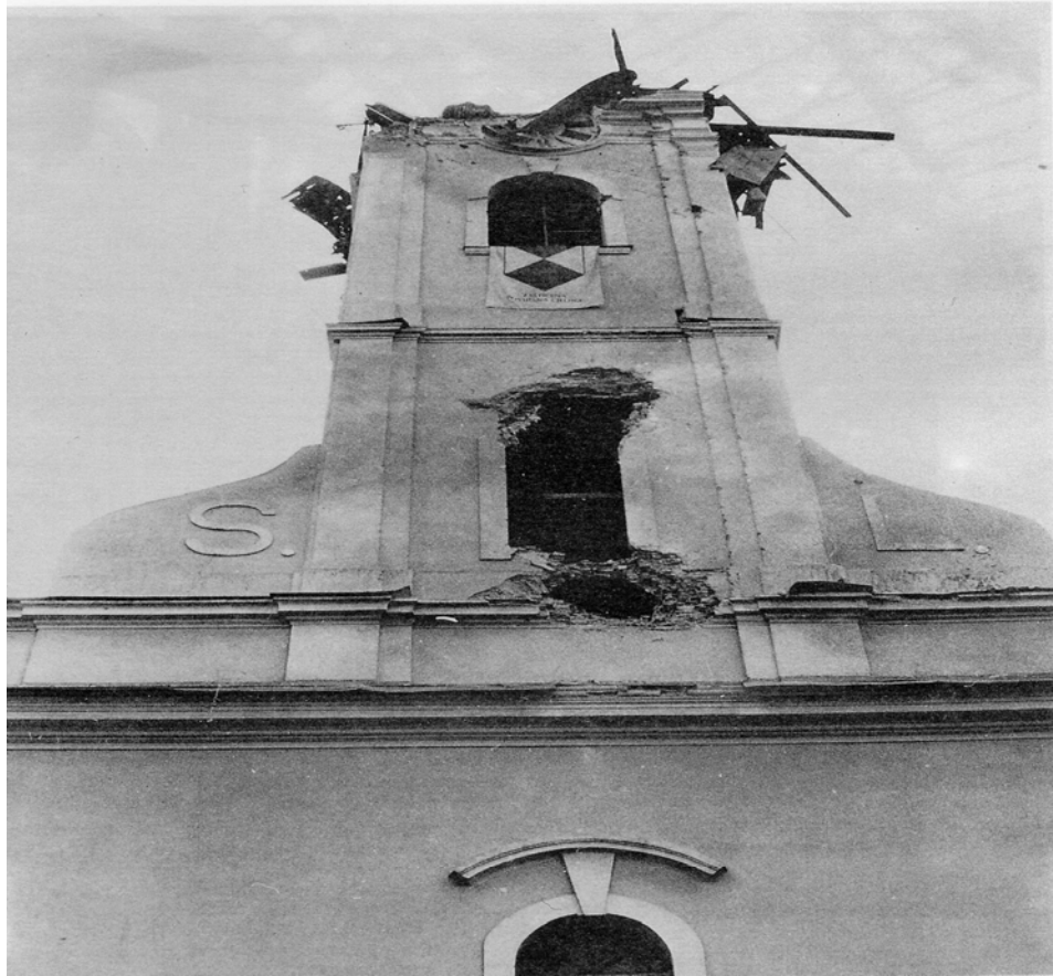
Croatia: The bell tower of The Church of St. Lawrence in Petrinja was struck during a bombardment despite the protective Blue Shield emblem of The Hague Convention flying from its window.
