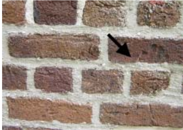
Figure 3:2 Exterior wall of Jerusalem Lutheran Church displays visible fingerprints in handmade bricks. (Source: author)
