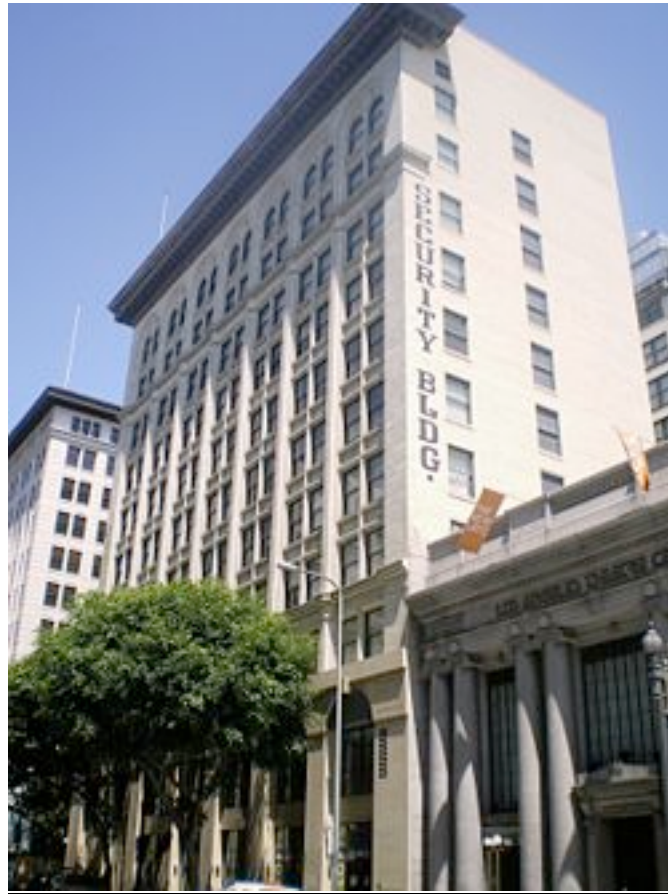
Figure 6-1: The Security Building 152
