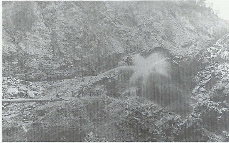
Hydraulic mining was brought to Georgia in the 1850s by miners returning from the California gold fields. A single miner using one of these giant water cannons could cut an enormous gash in a mountainside like this one on Crown Mountain just south of Dahlonega. This image was recorded about 1900 at the height of Georgia's short-lived second gold rush. Georgia Department of Archives and History.
