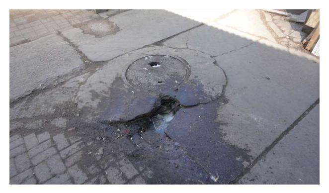
Figure 46. Wastewater gathered in broken pavement
