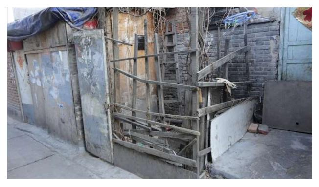
Figure 39. An illegal house built with wooden boards
