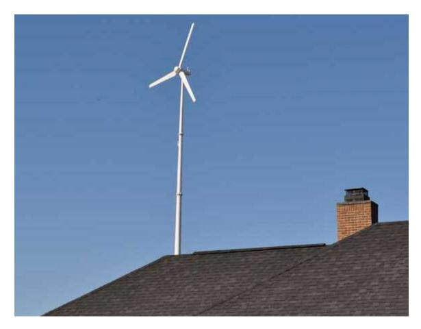
Figure 13. Building-mounted wind turbine (Front Generator Wind Turbine n.d.)
